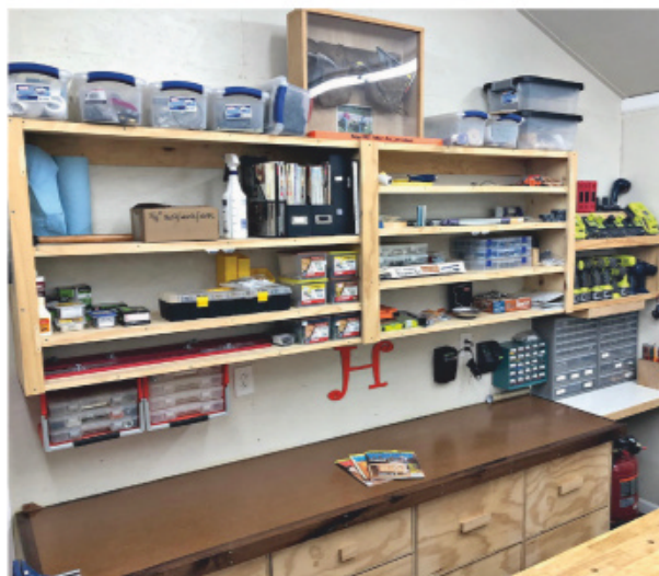
Walls lined with painted OSB provide a solid surface for attaching shelving and cabinets wherever needed.
