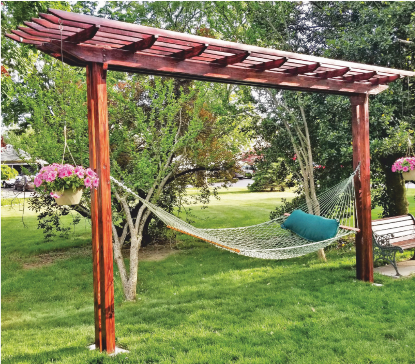
Rob Loeffler , of Pequannock, N.J., built the Double-feature Pergola, shown here in hammock-holding mode, from plans in issue 253 (May 2018). The stain is a home brew he came up with to match the adjacent ipe park bench.
