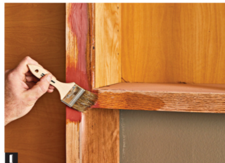
I Brush on two coats of lacquer. This seals the surface and allows you to peel away the veneer in the next steps should you need to reposition it.
