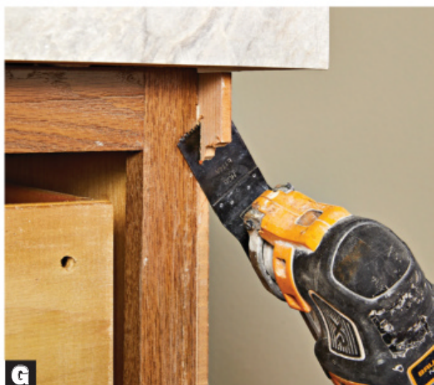
G Use a multitool or flush-cut saw to remove waste where the router can't reach.
