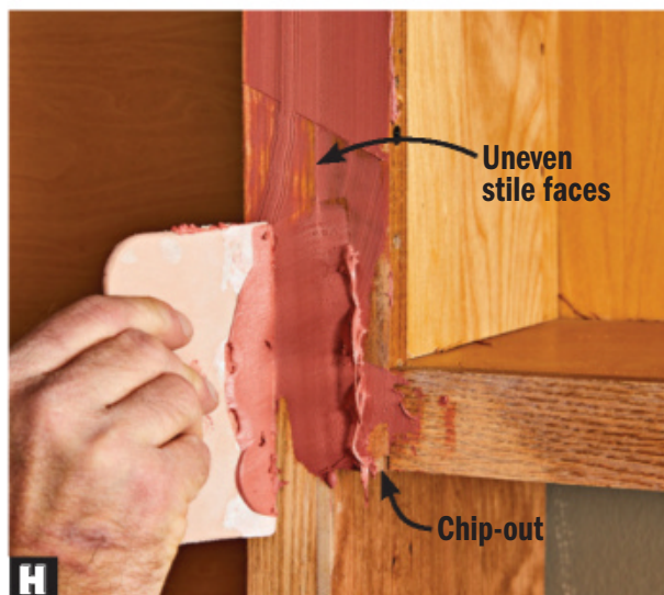
H An auto-body filler, such as Bondo, works well for filling imperfections and leveling surfaces. It cures quickly and sands easily.
