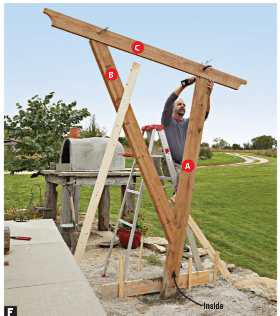
F Attach the beam to the A/B assembly with screws driven from the outside through the rabbeted ends into the beam.
