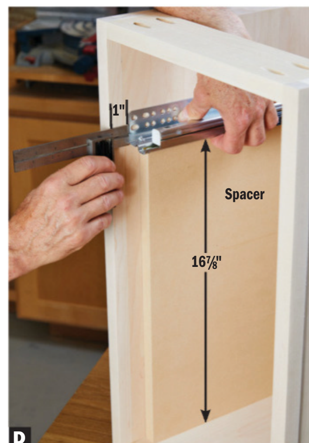
D Rest the upper slides on a spacer, position them 1" back from the pedestal front edge, and screw them in place.
