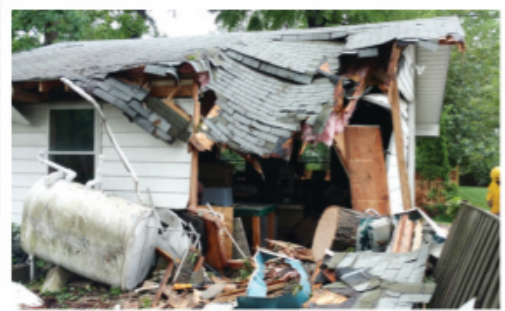
John Gunter's original detached garage workshop was destroyed by a tree during a wind storm (inset). He rebuilt on the existing foundation.
