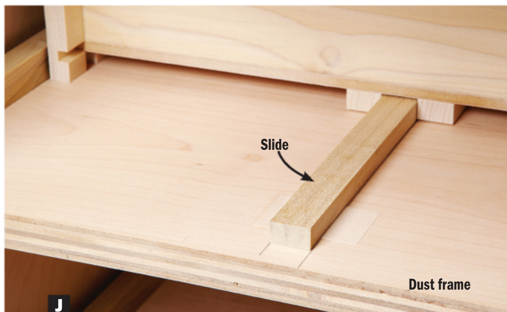
J A wood slide, such as this center-mounted version, keeps a drawer moving in a straight line front to back, and at a bargain price.
