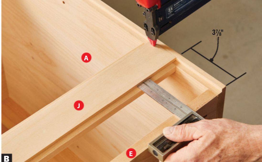
B Glue and nail the drawer-slide rail (J) to the lower-case sides (A).
