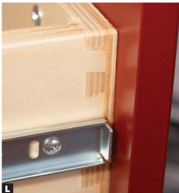
L This plywood drawer box with a painted false front functions well as a drawer, but lacks the perceived quality of a well-made solid-wood drawer.
