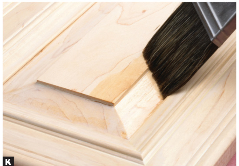
J Brushing contours with the grain causes runs and drips. Instead, brush with the profile, using thin coats from a lightly loaded brush.
