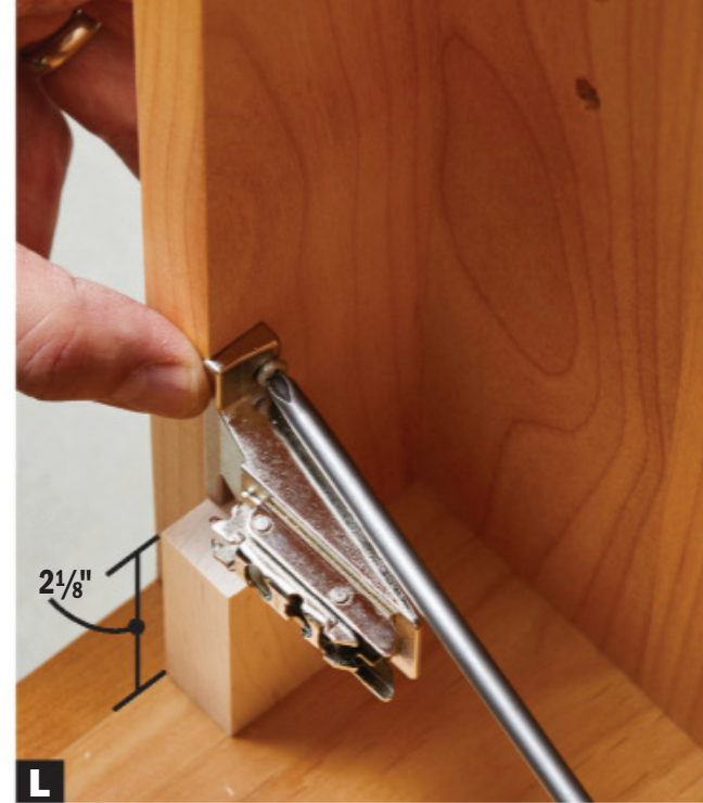
Screw the lower hinge-mounting plate to the face-frame stile, positioning it on a spacer resting on the case bottom.
