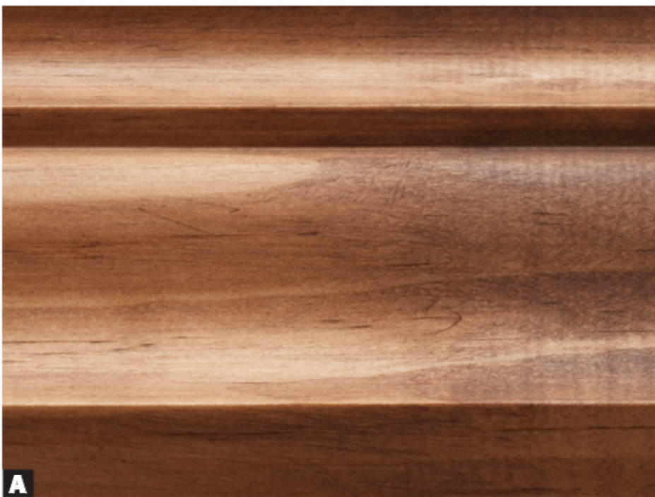
A The sanded molding section on the left takes stain evenly and shows no ridges, unlike the unsanded area on the right.
