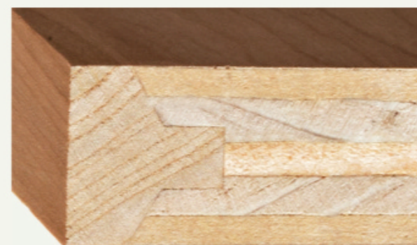
Thick tongue-and-groove edging
