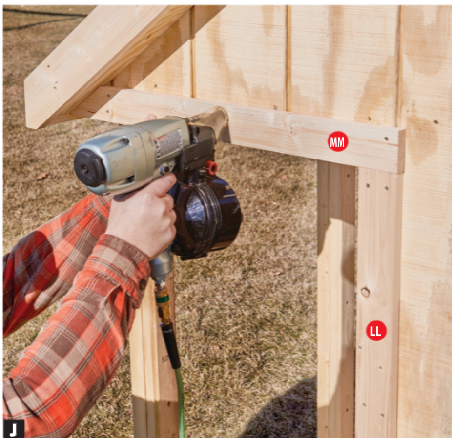
J Nail the overhang trim (MM) in place, covering the upper end of the front corner side trim (LL).
