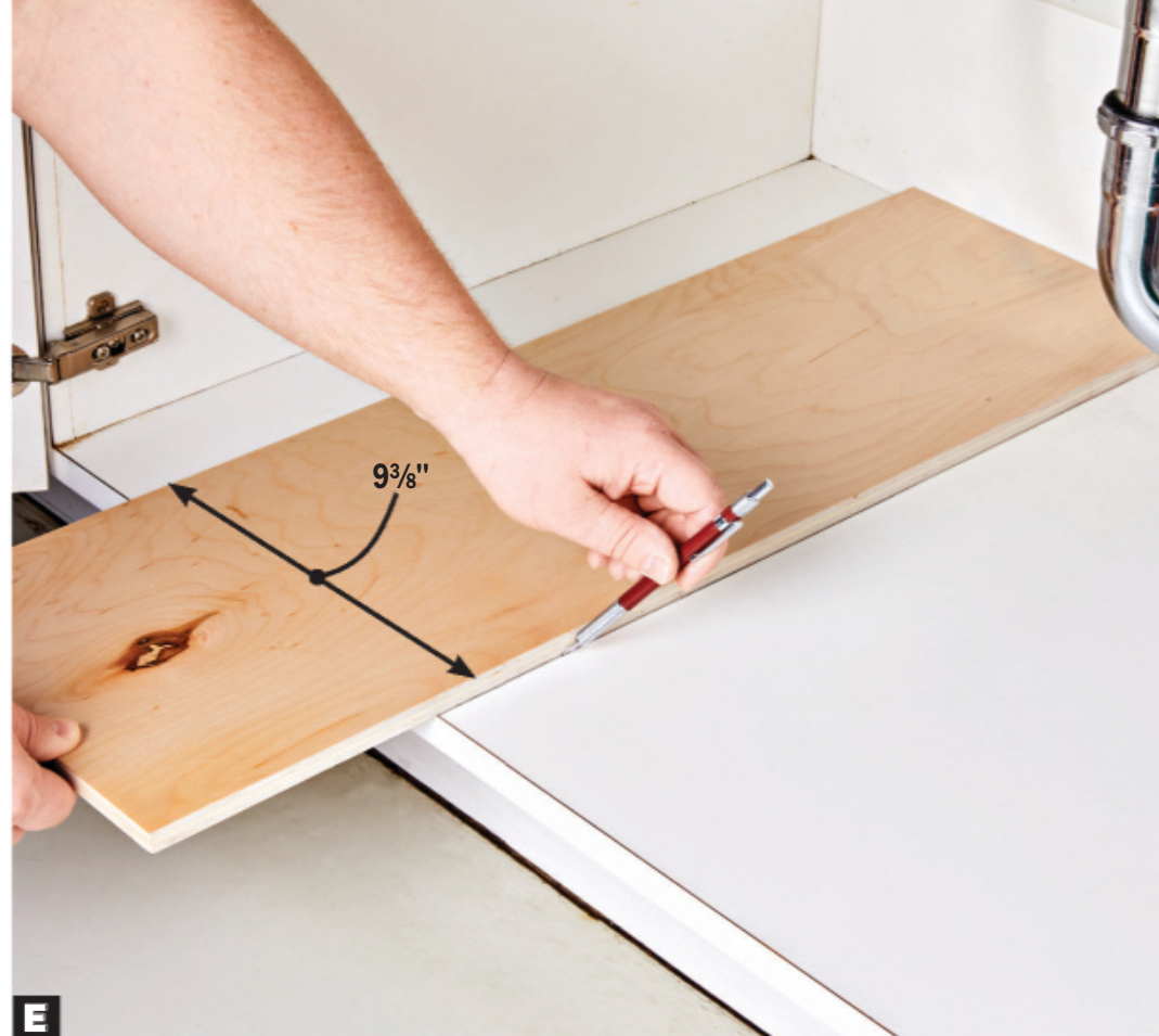
E Space centerlines 9 3/8" apart for slides on both the organizer and cabinet.
