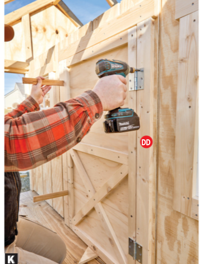
Insert shims to leave uniform gaps at the door top and sides and screw the hinges to the door side trim (DD).
