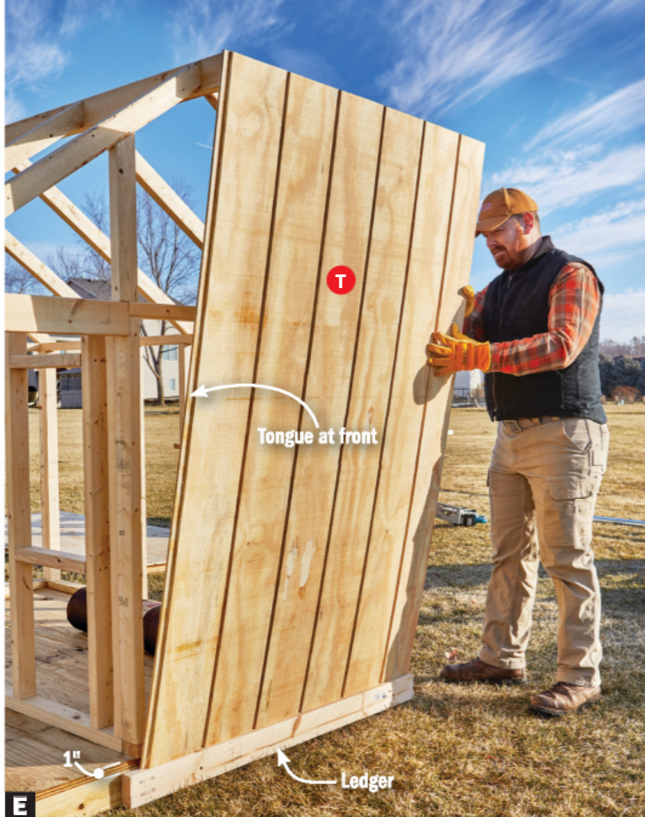
E Stand the end siding (T) on a temporary ledger screwed to the end joist 1" below the floor.
