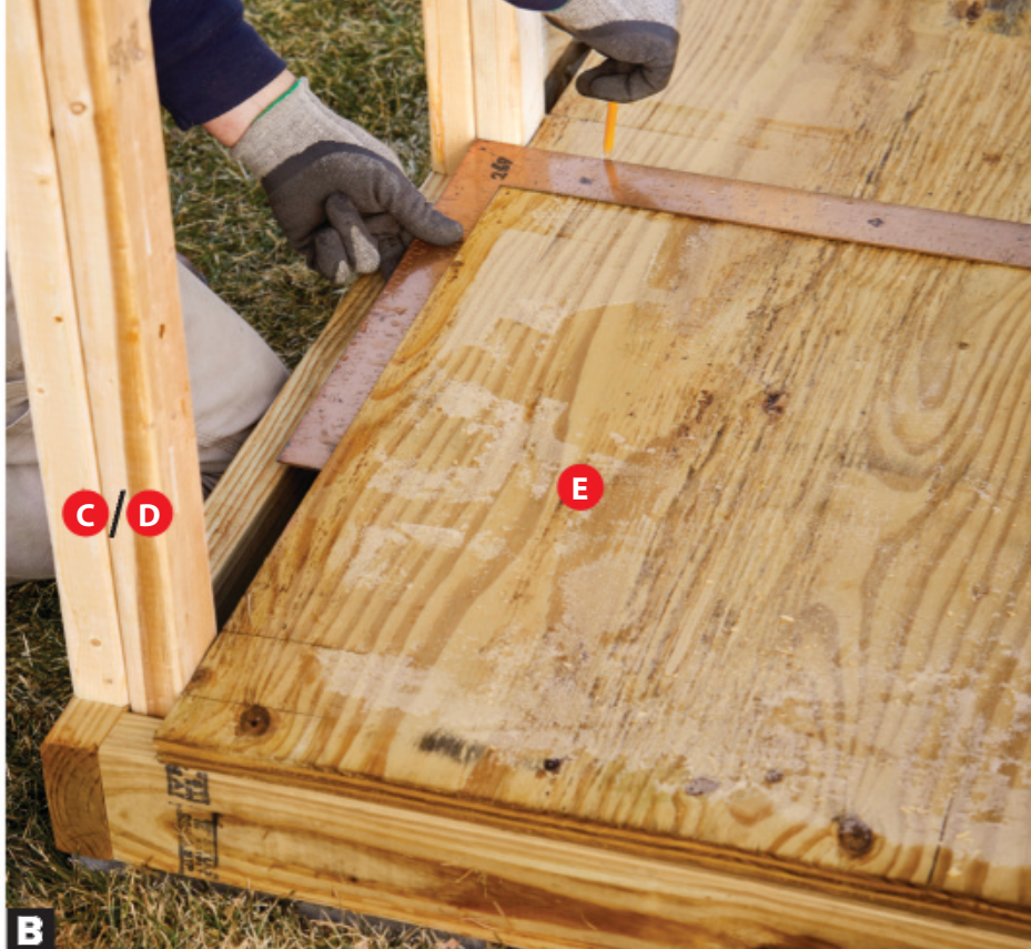
B Transfer the post (C/D) locations to the front floor panel (E) positioned on the floor frame flush at the ends.
