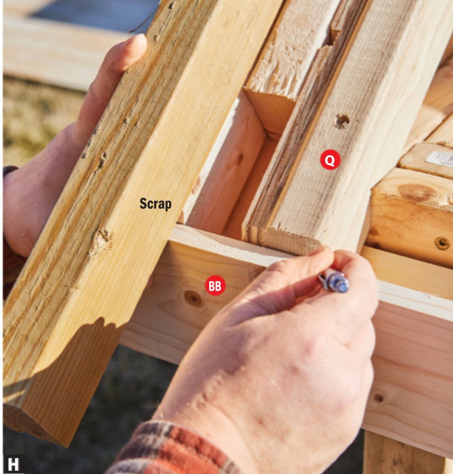
H Project the roof plane with a scrap 2x3, push the fascia (BB) against the underside, and mark the top edge of the fascia on the rafter (Q) ends.
