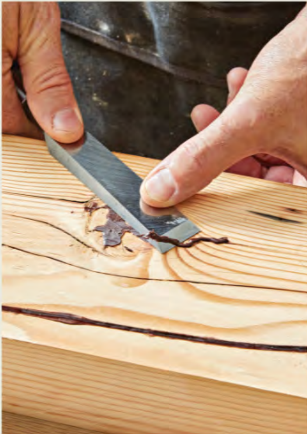
Pare excess glue flush with the surface. Do not remove excess glue with heavy sanding. The heat of sanding softens and smears the glue.
