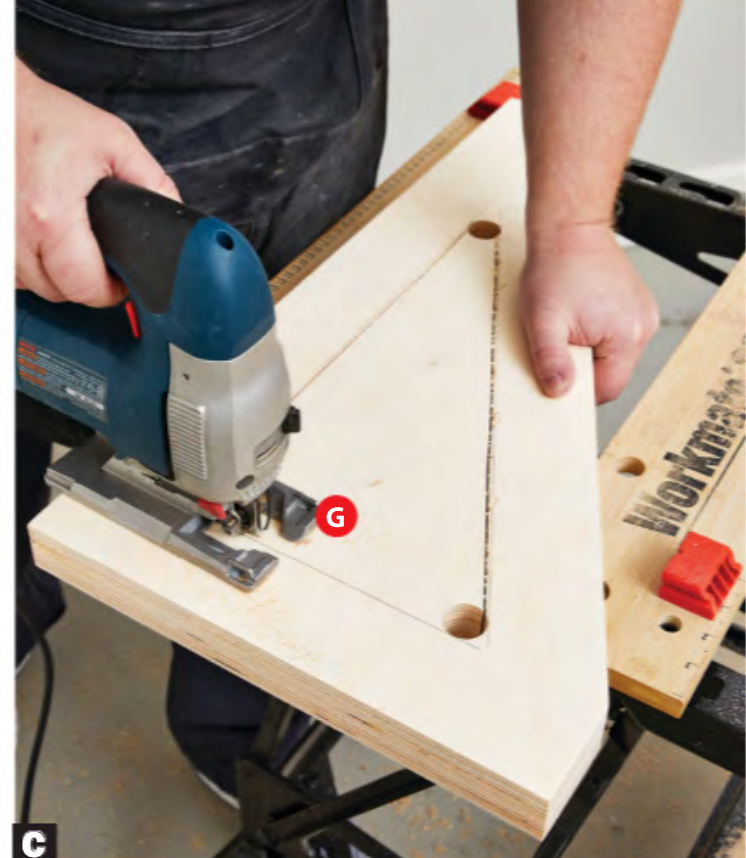
C Jigsaw on the waste side of the lines connecting the corner holes in the supports (G).
