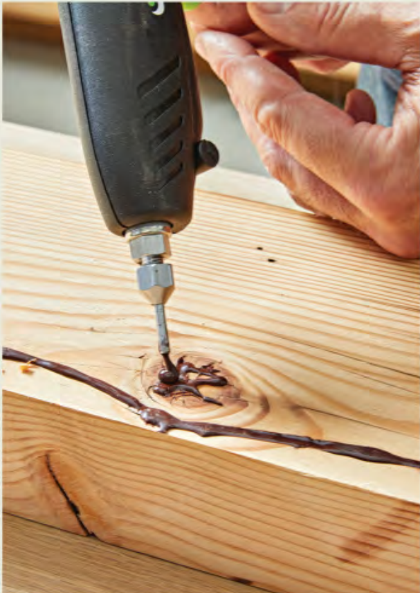
Inject hot glue into cracks and voids, gradually overfilling them. Allow the glue to cool fully.
