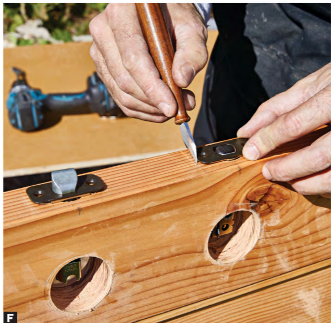
F Place the latch and bolt in the lockset holes and mark the mortises. Rout the mortises close to the marks with a trim router and mortise bit. Clean up the edges with a chisel.
