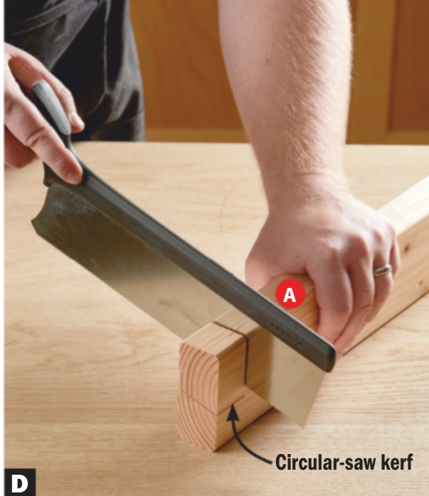
D Press a handsaw blade against the "keeper" side of the kerf and cut at an angle to remove the waste.
