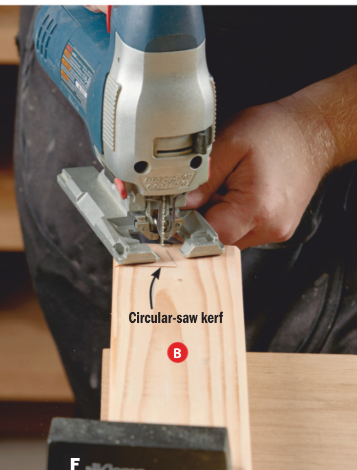
F Cut on the waste side of the scribed line connecting the end of the board to the circular-saw kerf.
