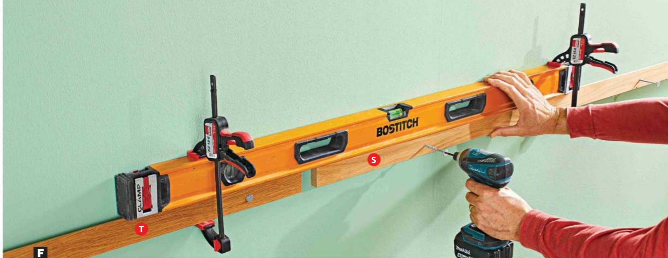
F Screw the cleats to the wall with 3½" screws. Drive screws into studs. Keep the tops of the three cleats level and even.
