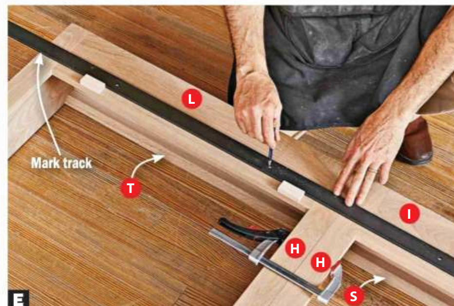
E Draw the track mounting holes on the cabinet face frames. Also mark the ends of the tracks flush at each side of the cabinets and identify each track for position.
