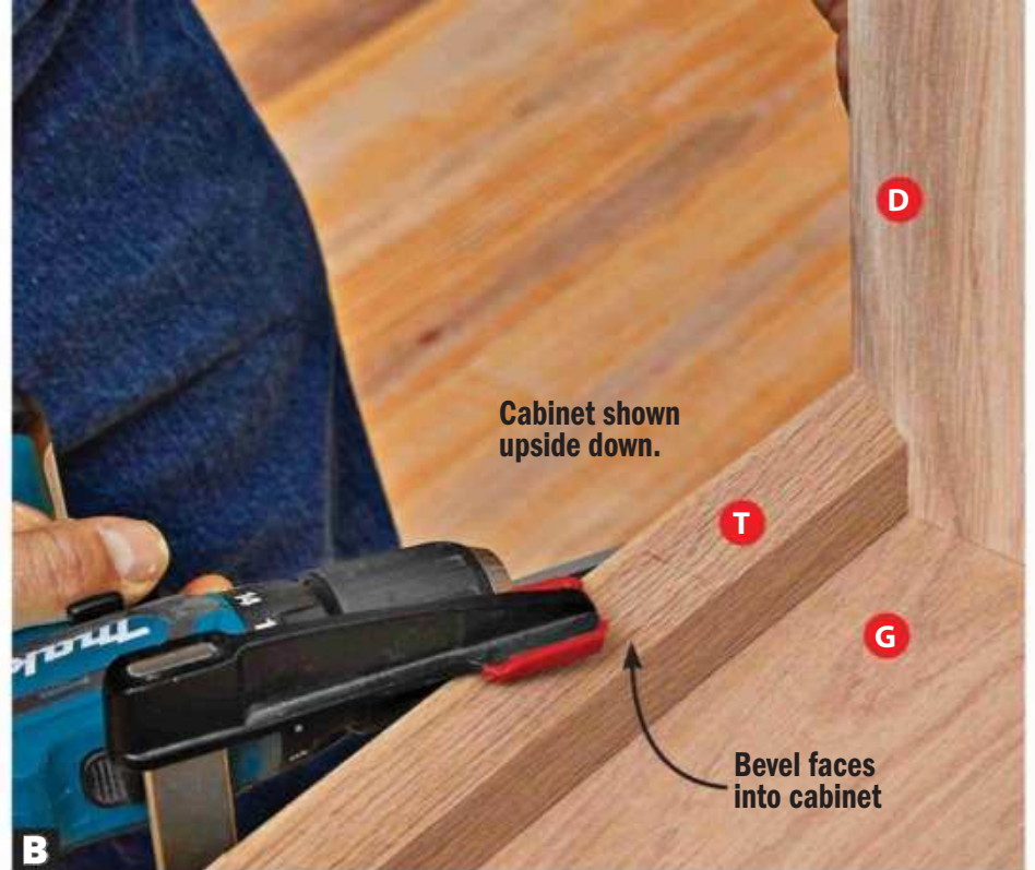
B Attach the beveled lower-cabinet cleats with pocket screws. The remaining beveled parts attach to the wall and mate with the case when you install the completed unit.
