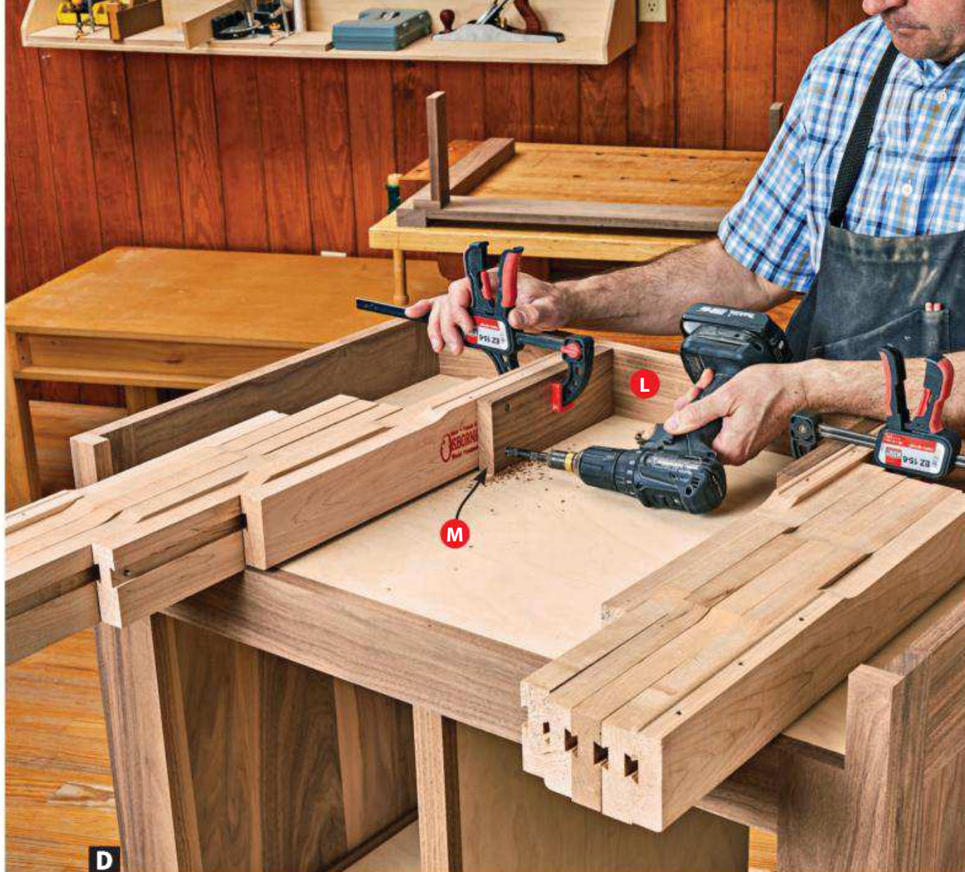
D Screw the table slides to the cleats (M) flush at the top, and with the slide ends against the back rail (L).
