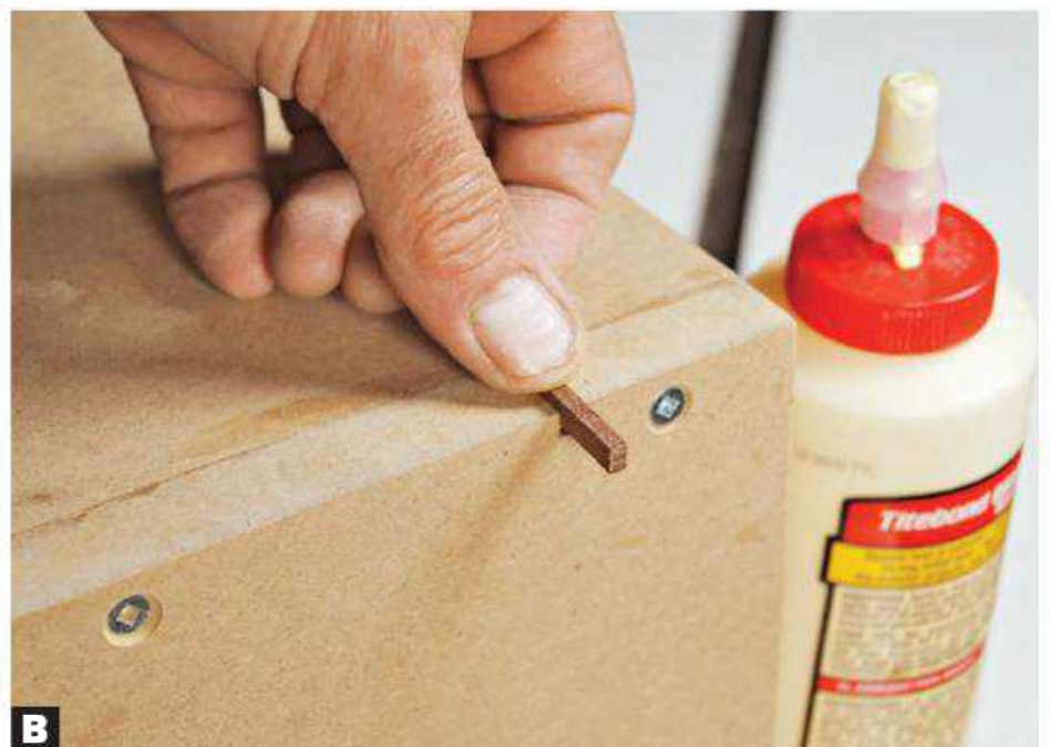
B Make a 1"-long hardwood key to fit the groove, and glue it in place.
