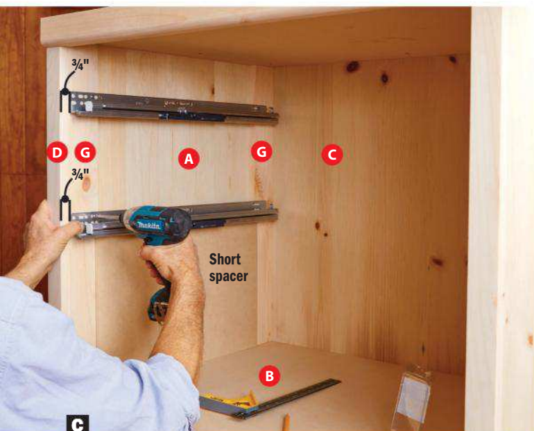
C A scrapwood spacer supports each drawer slide parallel with the cabinet bottom while you screw it in place.
