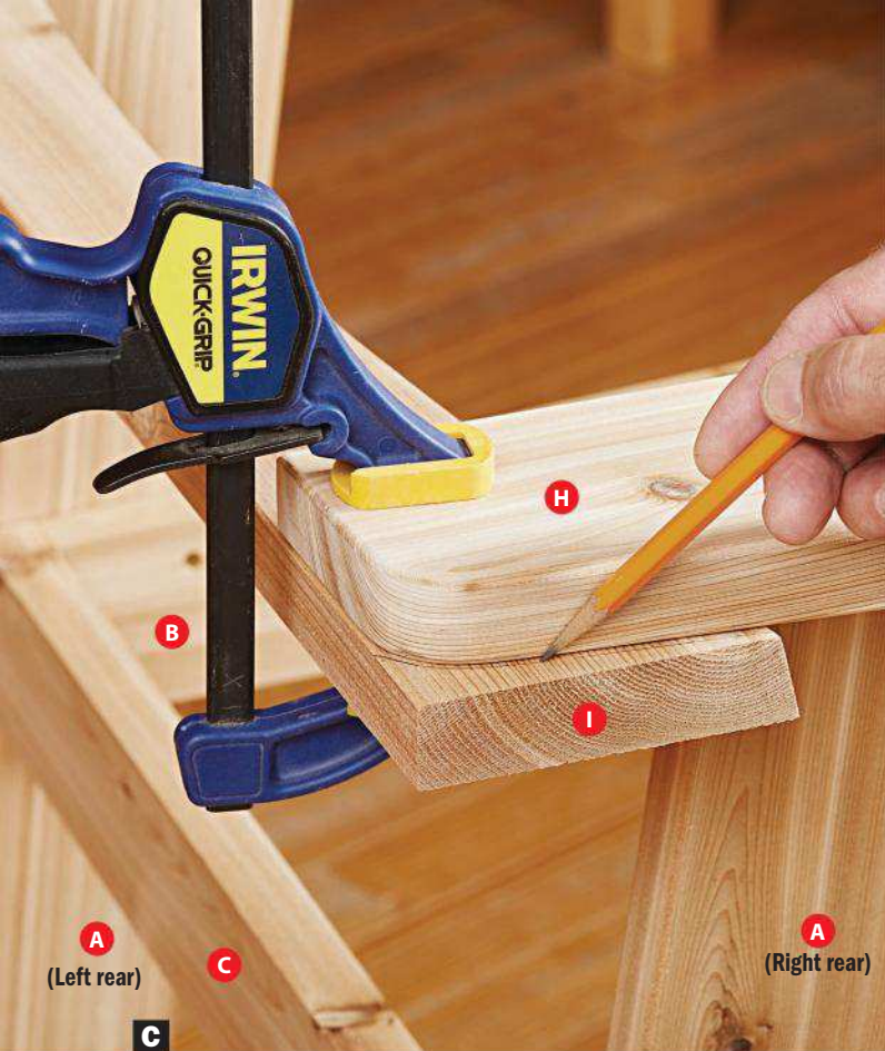
C Mark the curve at the back of each arm (H) on the backrest upper rail (I). Cut the ends of the rail, screw and glue the part in place, and sand the ends flush with the arms.
