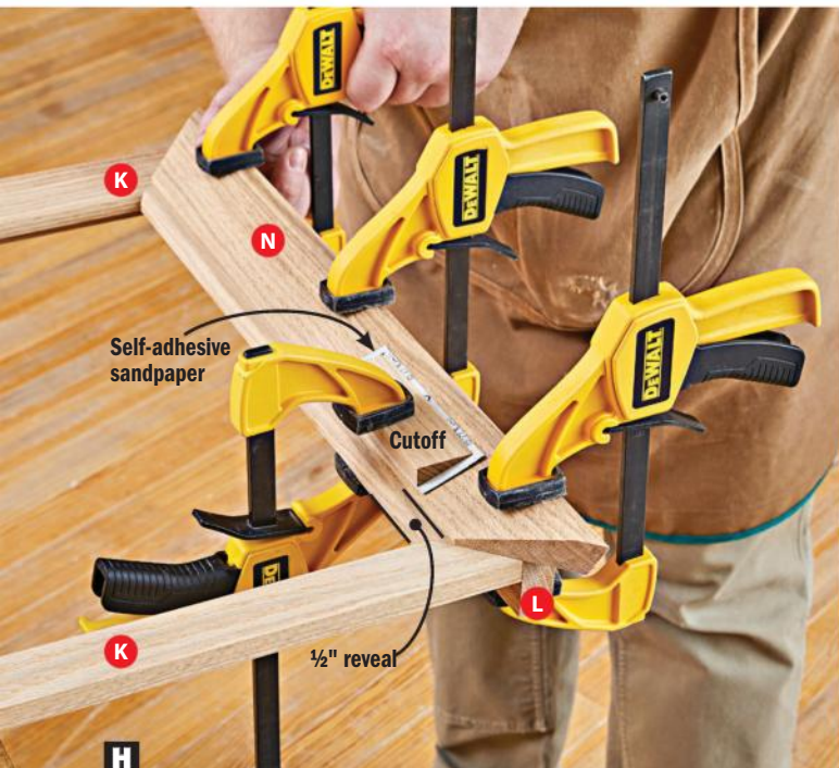
H Glue the moldings in place, maintaining a 1/2" reveal around the opening. Tip! Attach self-adhesive sandpaper to scraps of bevel-cut stock to make effective clamp blocks.
