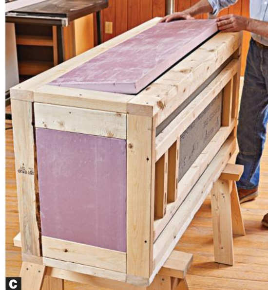
C Cut foam insulation board to fit snugly between the framing members and secure it with construction adhesive.
