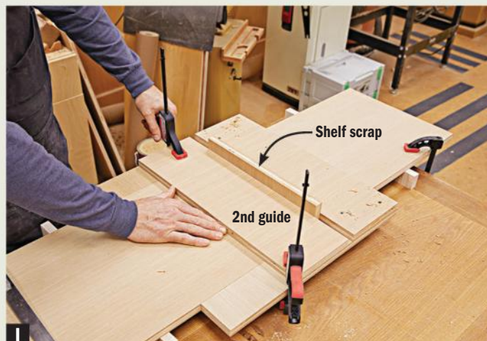
I Place a scrap of shelf stock against the first guide, position the second guide, and clamp it in place. The scrap should fit without play but be easy to remove. Screw on the second guide.
