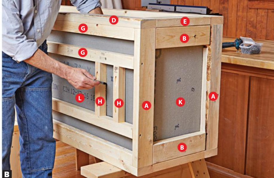
B Hold the back panel against the framing and mark the vent openings. Drill \frac{1}{4} " start holes and make the cutouts using a jigsaw with a metal-cutting or carbide-edge blade.
