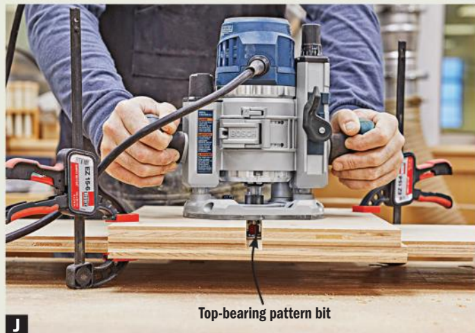
J Align the edge of one guide with the dado-layout mark and clamp the jig in place. Rout the dado in two passes with a top-bearing pattern bit.
