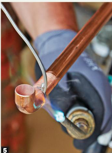
5 Using a torch, heat the joint. When flux bubbles out, touch solder to the joint. As the solder melts, capillary action sucks it into the joint. Be sure to apply solder all around the joint.
