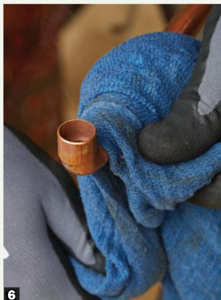
6 When finished, wipe off excess flux, which can corrode the pipe over time. Allow the pipe to cool before installing.
