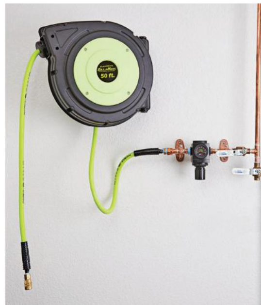
A hose reel makes for easy hose management at a drop. You can buy a reel with a swivel mounting bracket so it stores flat against the wall when not in use.
