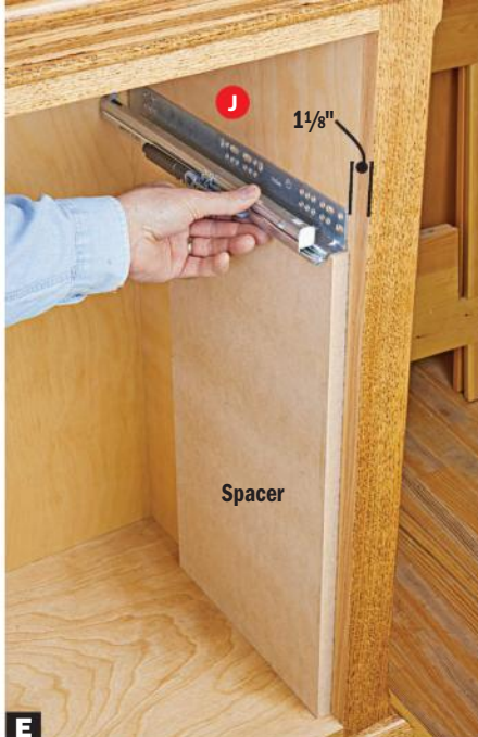
E Rest the cabinet member of a drawer-slide on the spacer. Screw the slide to the liner (J). Repeat on the other side.
