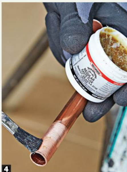
4 Apply flux to the pipe end as well as the fitting. Slide the fitting onto the pipe, making sure to align it as needed to correspond with other fittings already installed.
