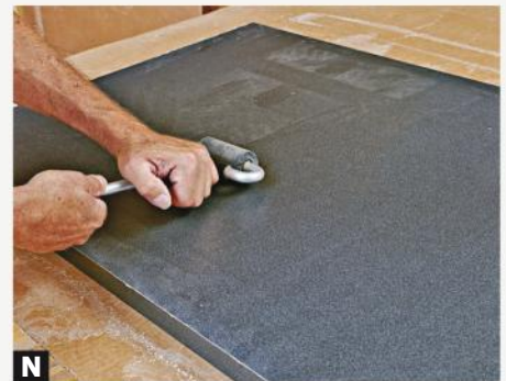
N Firmly press the laminate onto the countertop using a roller, working over the surface across the width and along the length. Pay special attention to the edges.
