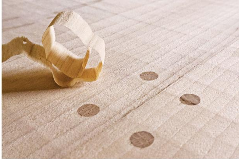
If the glue line should open up , the pinned tenons keep the joint together, while allowing enough give for the timber's seasonal movement. And they look rather fetching.
