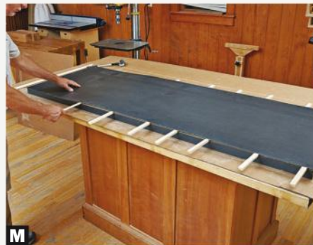
M Starting at one end, withdraw the scrapwood strips one at a time as you press the laminate onto the countertop, smoothing it from side to side with your hand.
