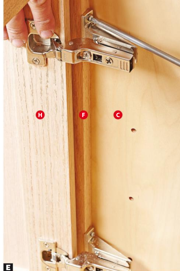
E Finish the hinge installation by snapping the lower hinge onto the lower hinge-mounting plate, positioning the upper mounting plate against the face-frame stile, and screwing the plate in place.
