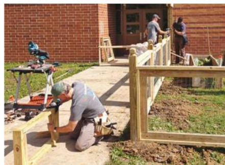
On-site, design editors Kevin Boyle and John Olson assemble the gate (background), while deputy editor Craig Ruegsegger custom-builds the final fence panel to fit (foreground).
