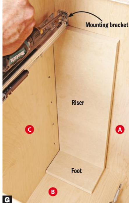
G Attach the back of the slide by screwing the rear-mounting bracket to the cabinet back. Do not make any side-to-side adjustment.
