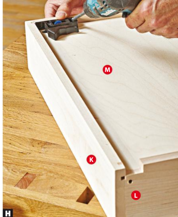
H Position the drawer-slide mounting clips in the bottom front corners of the drawers and screw them to the drawer fronts.
