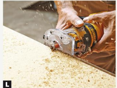
L Trim the edge strips flush with the countertop using a bottom-bearing flush-trim router bit. Adjust the bit to expose \frac{3}{32} " of the cutters below the router base.
