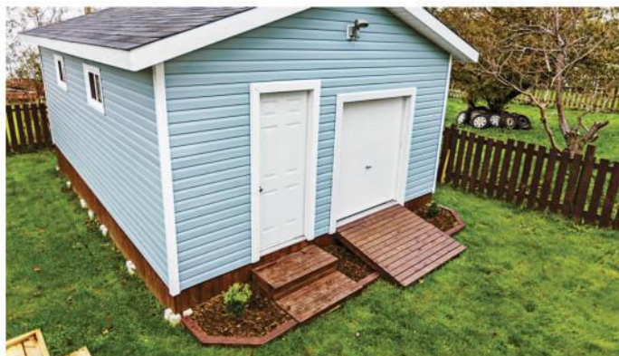
The 5x6' overhead door and ramp of Mike Hayes' 16x24' shop make it easy to move equipment and materials in and out.
