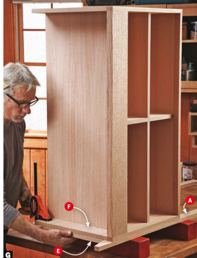
G Align the drawer case side (F) with the bottom edge of the side bottom rail (E). Bring the front of the case flush with the front edge of the leg (A).
