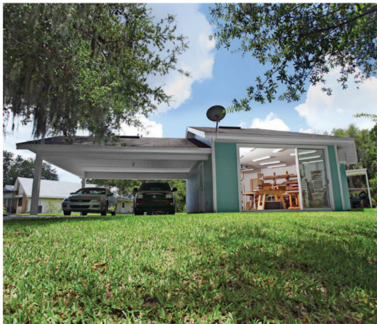
An extension of his double carport, Dave's shop features sliding door panels perfect for letting in plenty of Florida's sunshine and fresh air.
