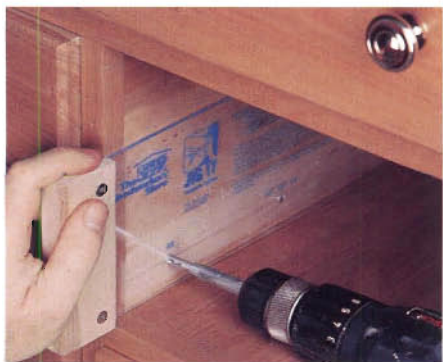
Figure 8: Try this specially designed jig (available from The Woodworkers' Store, 1-800-279-4441) to install the drawer slides correctly.
