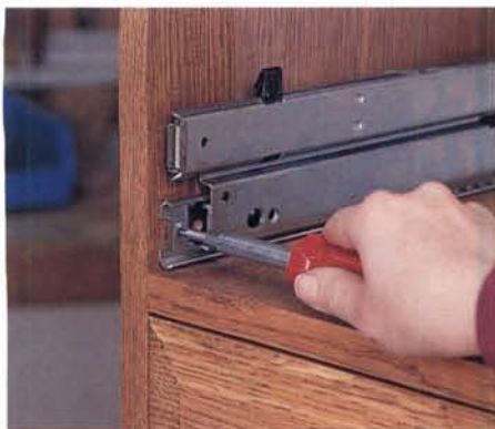
Figure 4: Install the large component of each slide 3/8" from the front edges of the cabinet so the drawer faces can sit flush in the openings.
