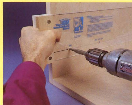
Once you determine the drawer spacing, hold the Jig-it to your marks and drill the pilot holes.
