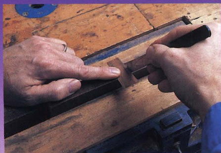
Step 4: After chopping the second edge of the patch at a small angle, push the patch in the hole and transfer this angle to the rail with a knife.
