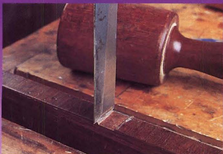
Step 1: Begin cleaning up the hole where the piece is missing from the rail by straightening one of its edges with a sharp chisel.
