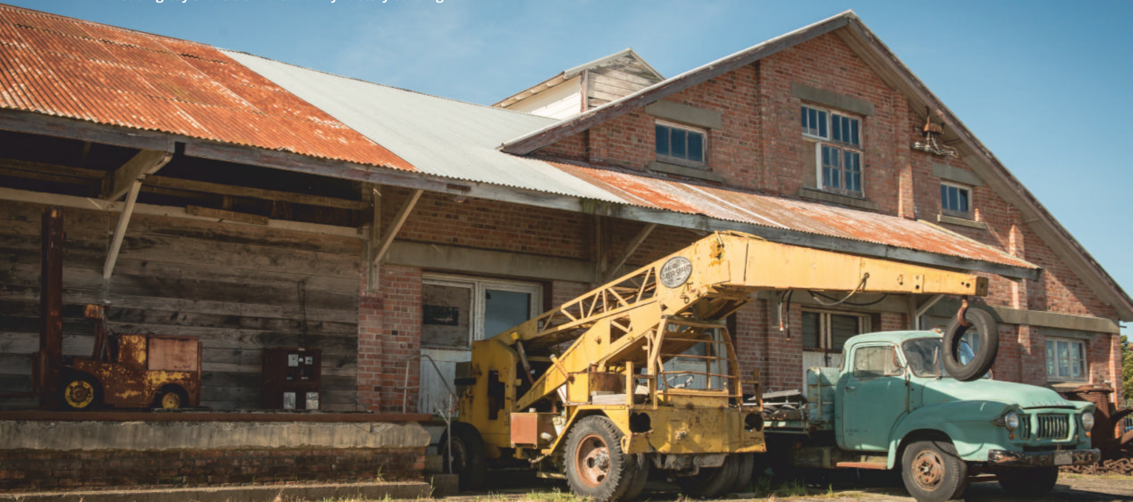
Loading bay of the old Kia Ora Dairy Factory building
