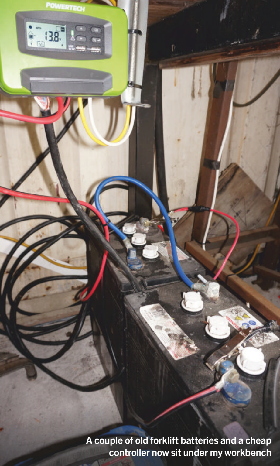
No. 2 battery bank: 201-amp-hour, 2V cells
