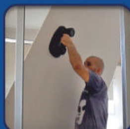
Wall and Tile
