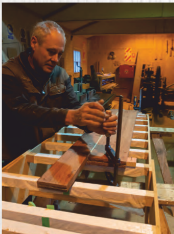
Cramping a sill onto a curved jig
