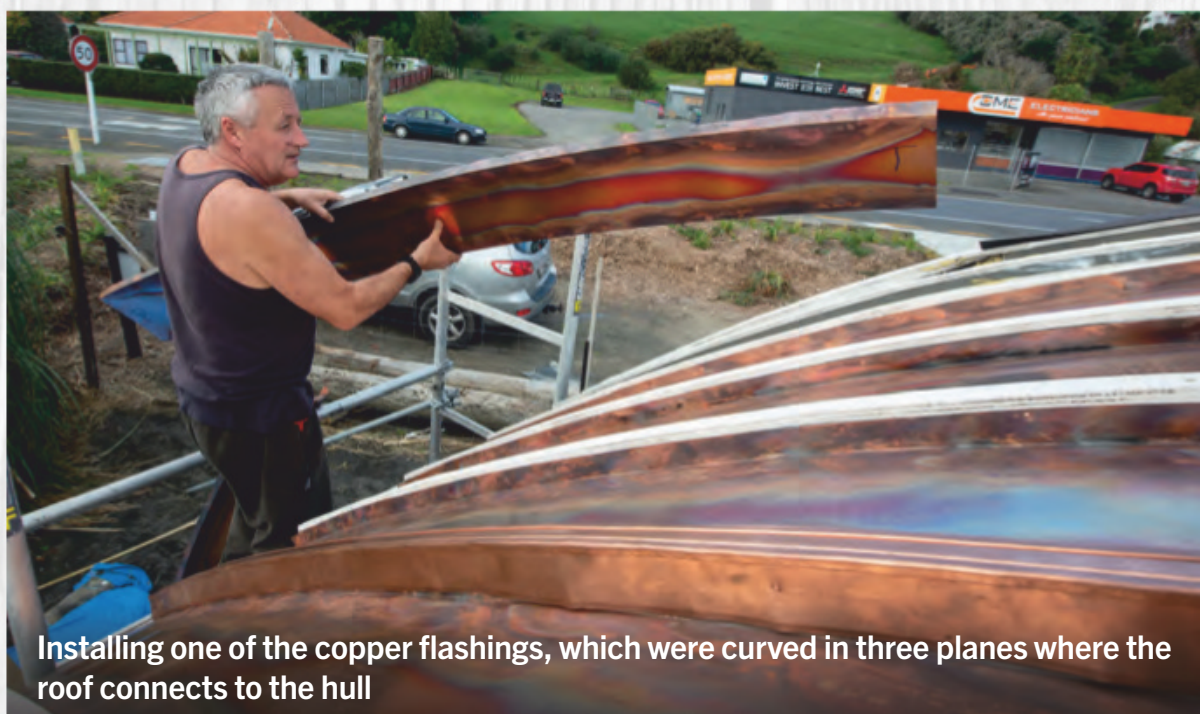
View of the end of one of the curved roof pieces showing the three-piece flashing system
