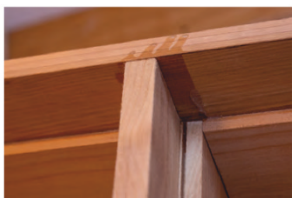
Setting out a mortice & tenon joint on one of the windows
