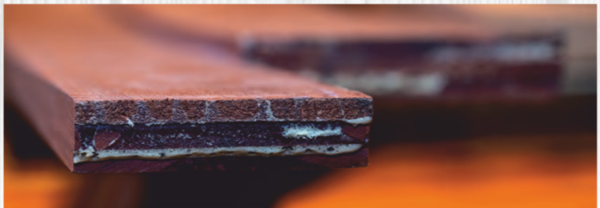
End shot of a finished sill showing the laminations in jarrah and polyurethane gap expanding foam glue, yet to be cut to finished dimension
