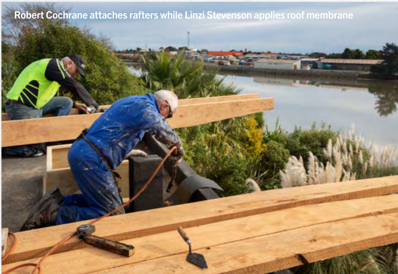
Keith Turner prepares the rainscreen battens
