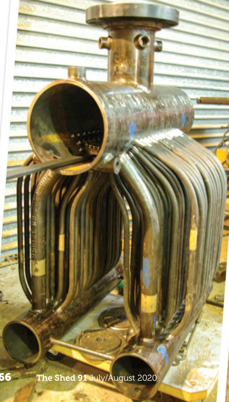
Building the boiler
