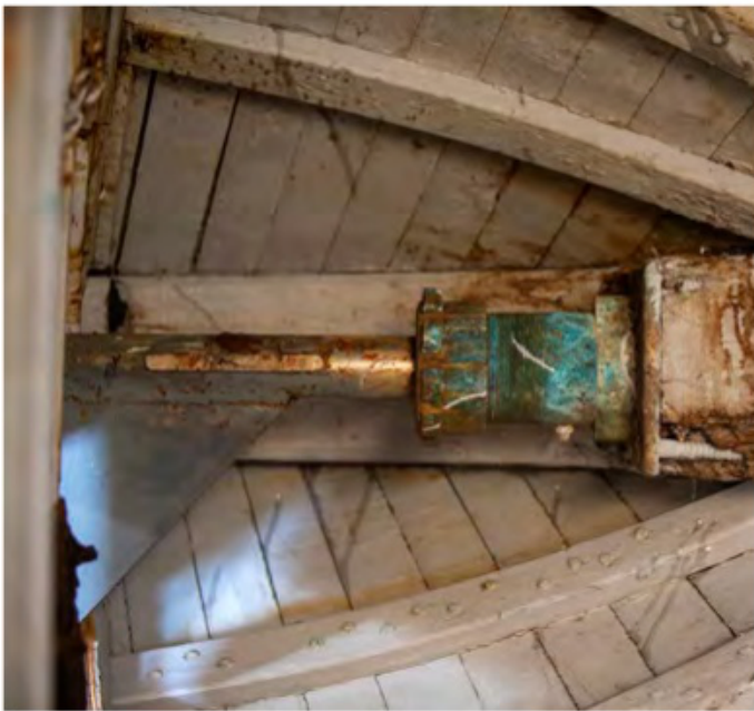
The old rudder stock is visible on the left, now connected structurally to the new building via Mike’s wide steel gusset.
