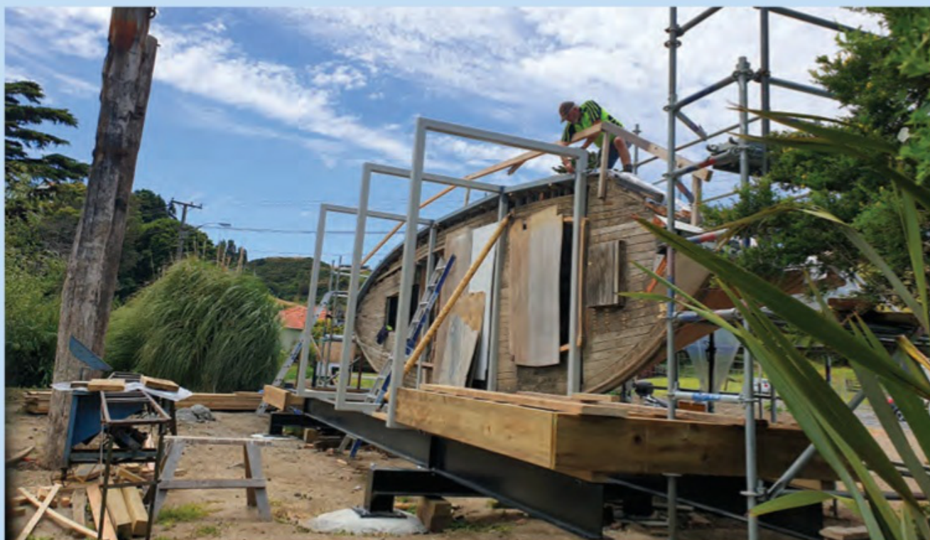
Robert attaches plastic sheeting to the outside of the hull to aid drying out in the early stages.
