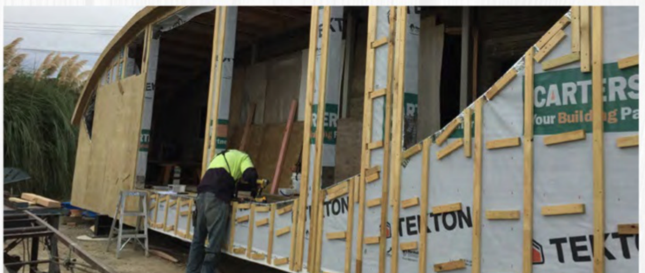
The new exterior façade batted out ready for a plywood skin which will form the base façade under the rainscreen.
