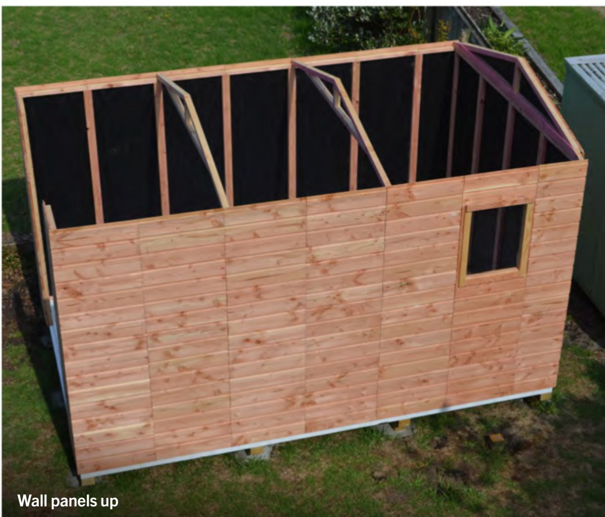
Wall panels are stood up on the edge of the floor frame and screwed to each other
