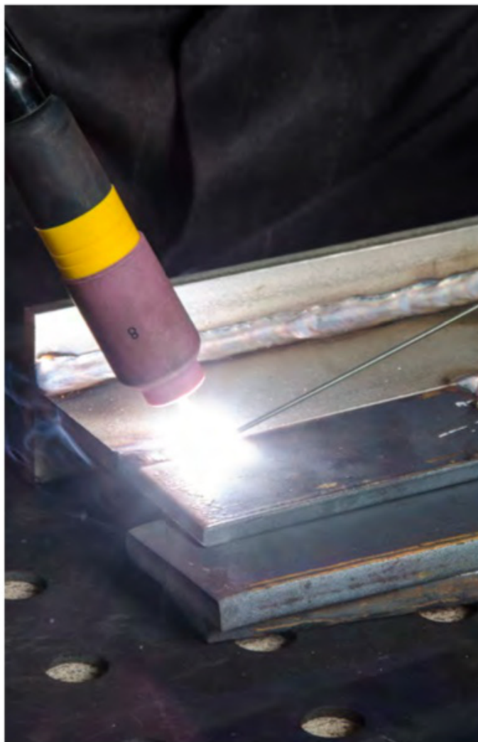
TIG welding stainless to mild steel
