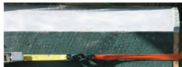
Boxing uses tie-down for the slab pour. The slab is 20mm deeper than the slab in the original article
