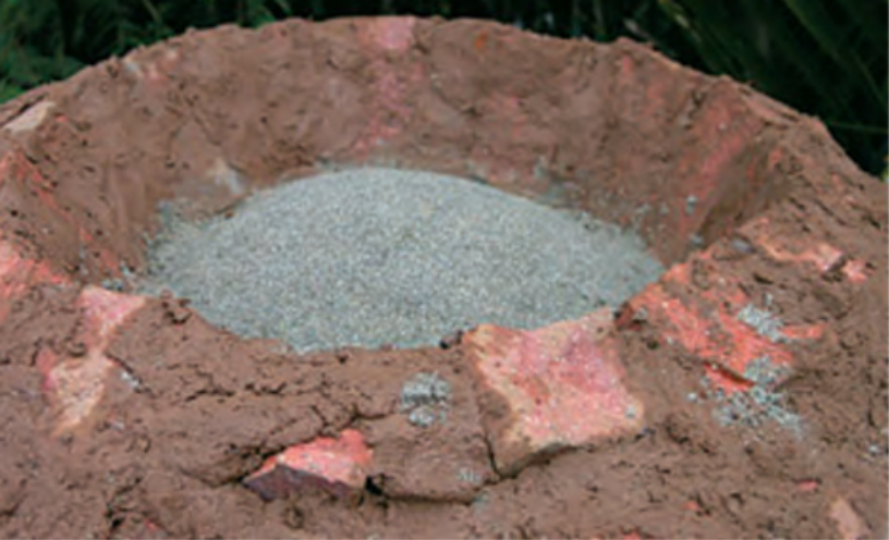
Cover the exposed crown of the dome support with dampened sand
