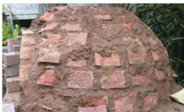
The dome in progress
