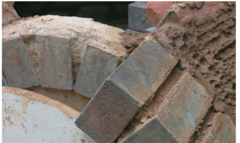
The outer arch uses whole bricks on a plywood former with a 325mm radius
