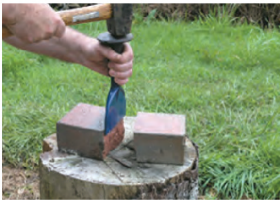
Cutting the bricks in half. Half bricks are used throughout the dome
