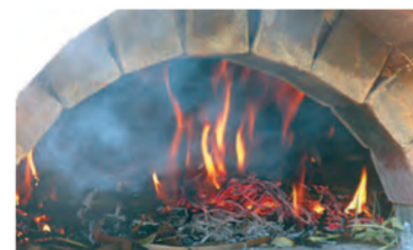
Drying out the fire with a smoke circulation test
