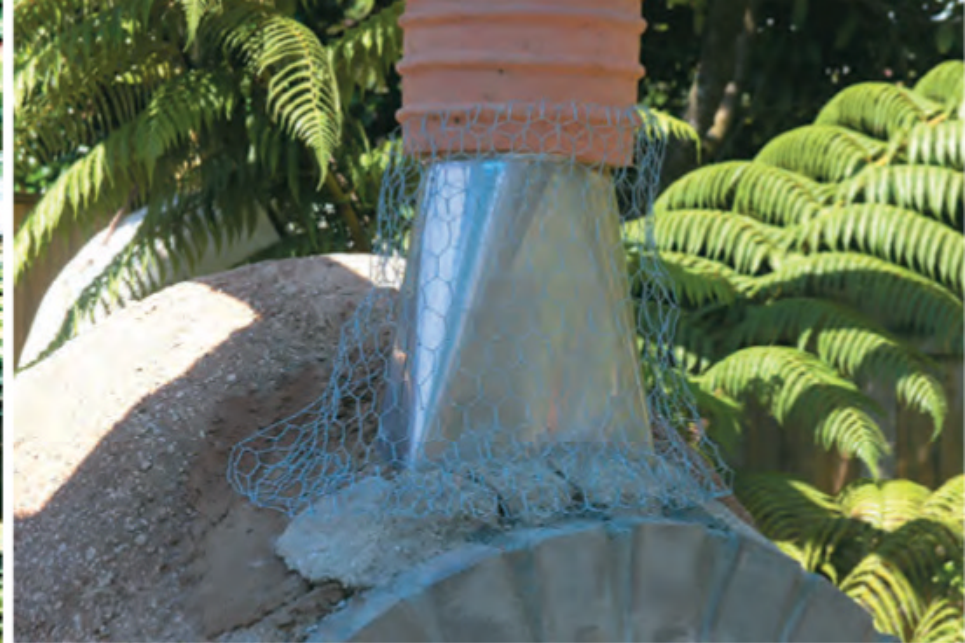
The space between the chicken mesh and flue allows for expansion
