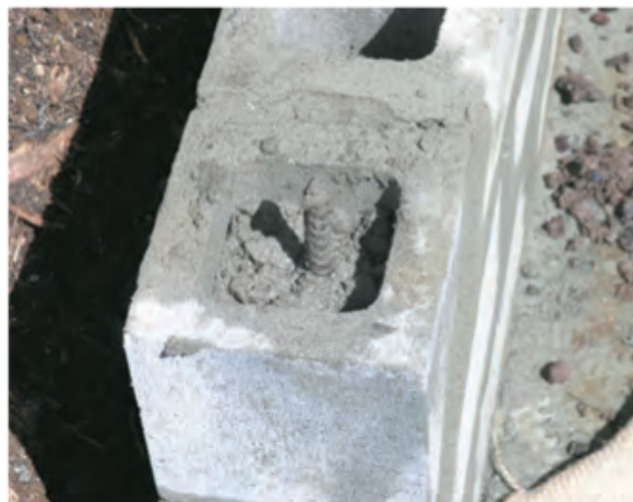
Rebar in corners
