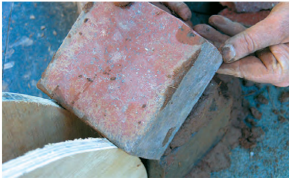
The inner arch uses two plywood semicircles as a form
