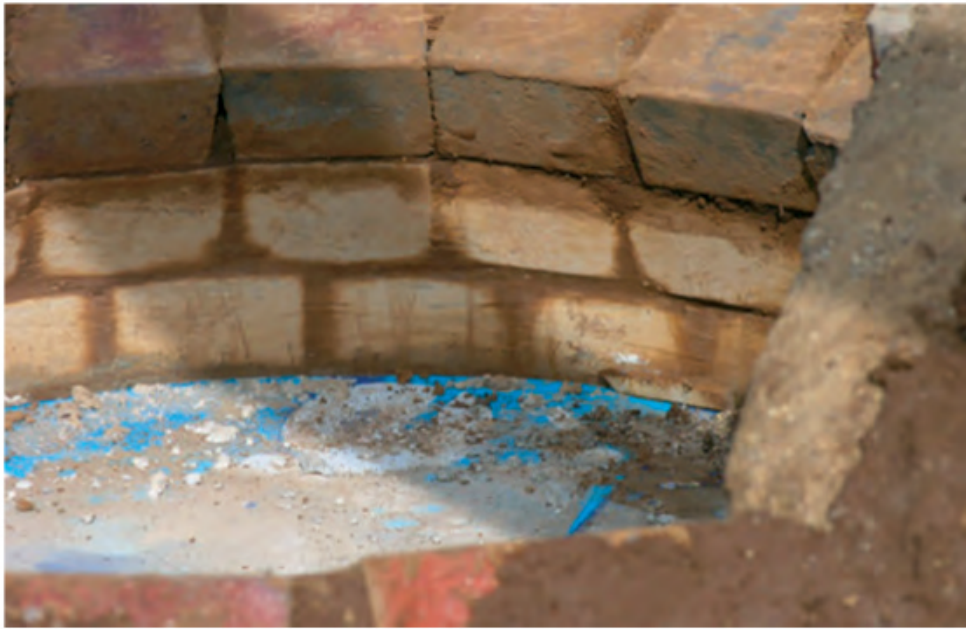
First courses of bricks. Note the blue plastic sheet protecting the oven floor
