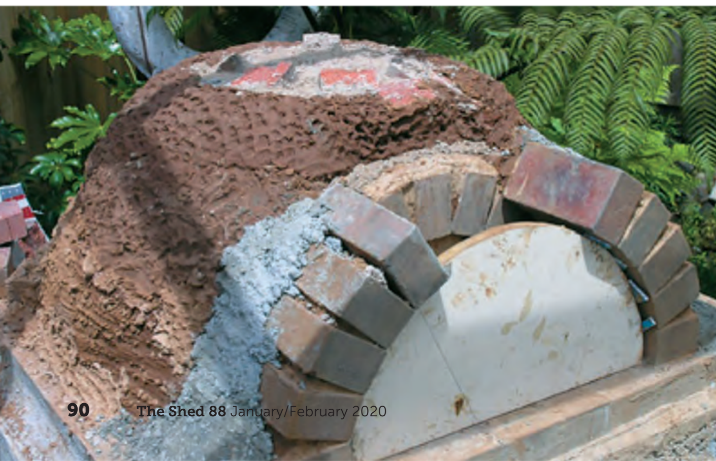
Over the arch, lay a mix of refractory concrete like a collar to key the bricks together. Note the dome bulked out with broken bricks
