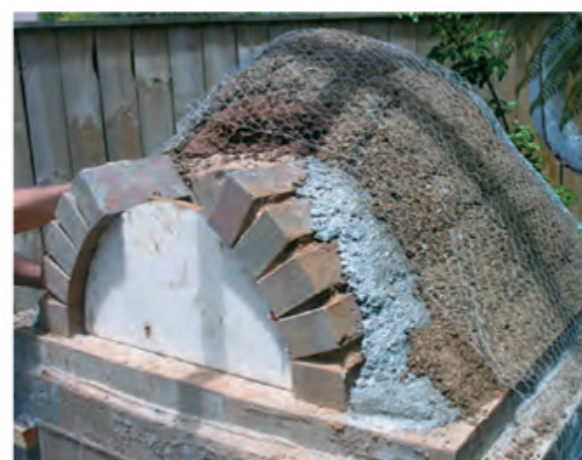
Chicken wire over the insulation layer provides a key for the render coat to adhere to. Note gap at the front for the flue
