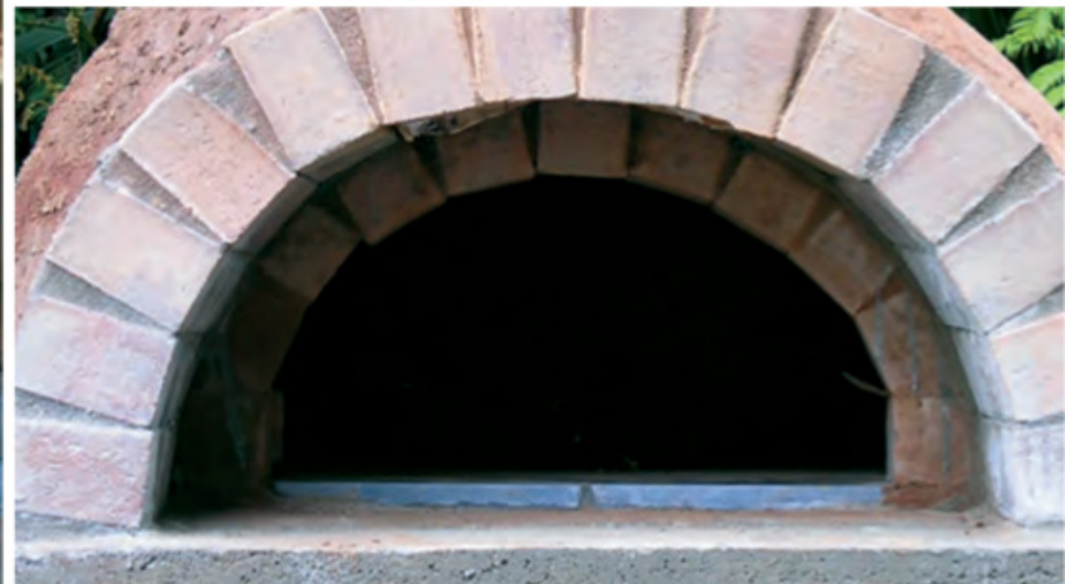
Inner arch to support the door
