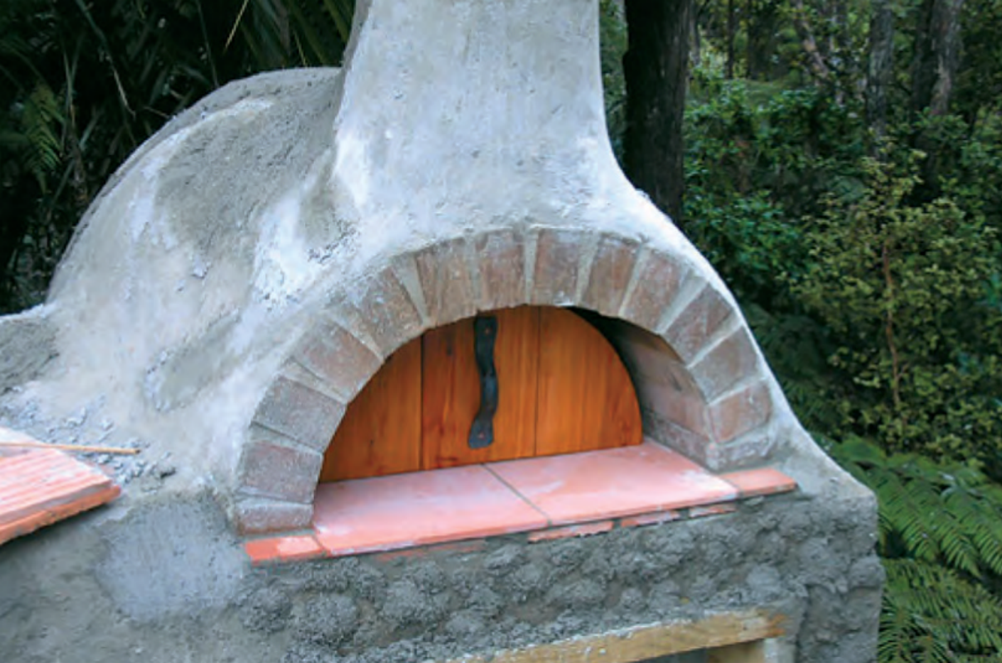
The door cut to shape and terracotta tiles on the entrance sill for the finishing touch
