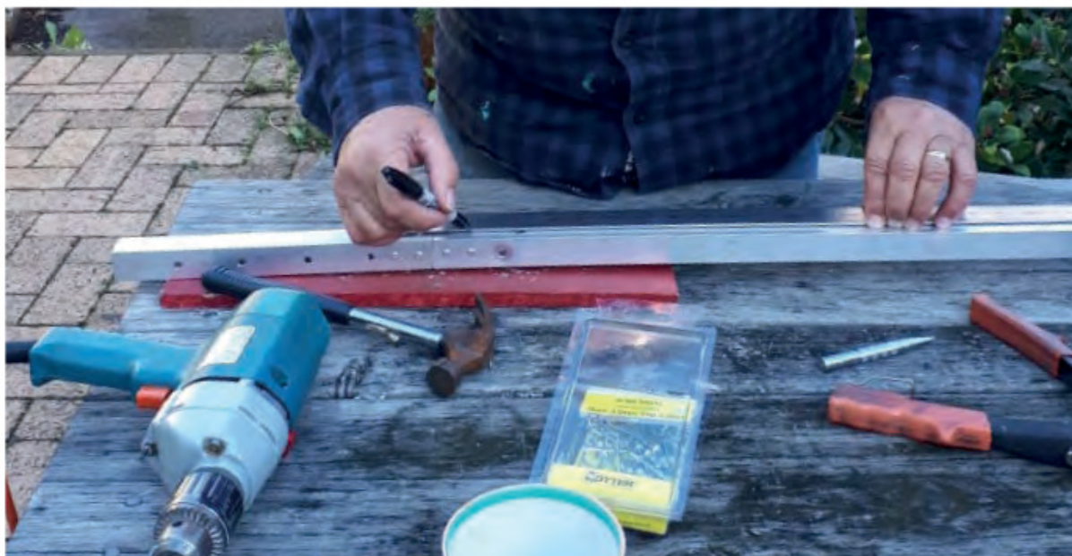
Above: Kathy's husband Pete installing one of the extensions
