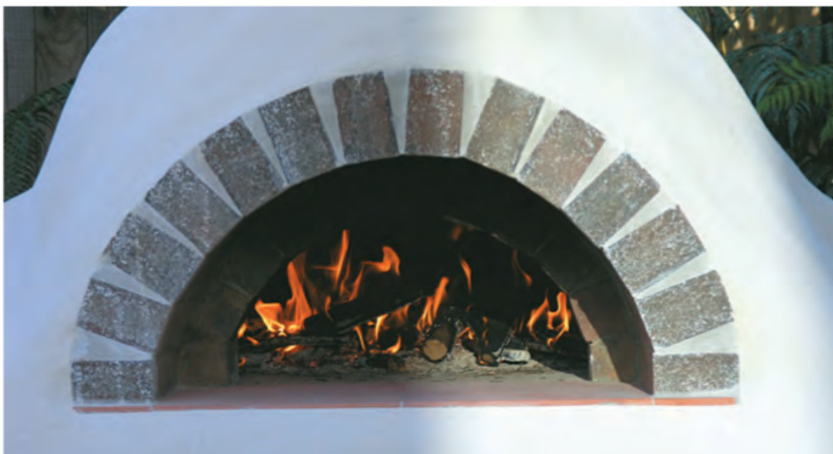
Lime/sand/cement render finishes another oven
