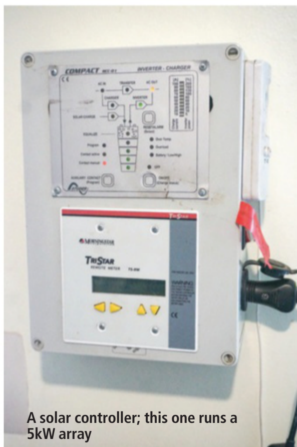
Solar controller (white, centre) and inverter (right). This is an off-grid 230V set-up
