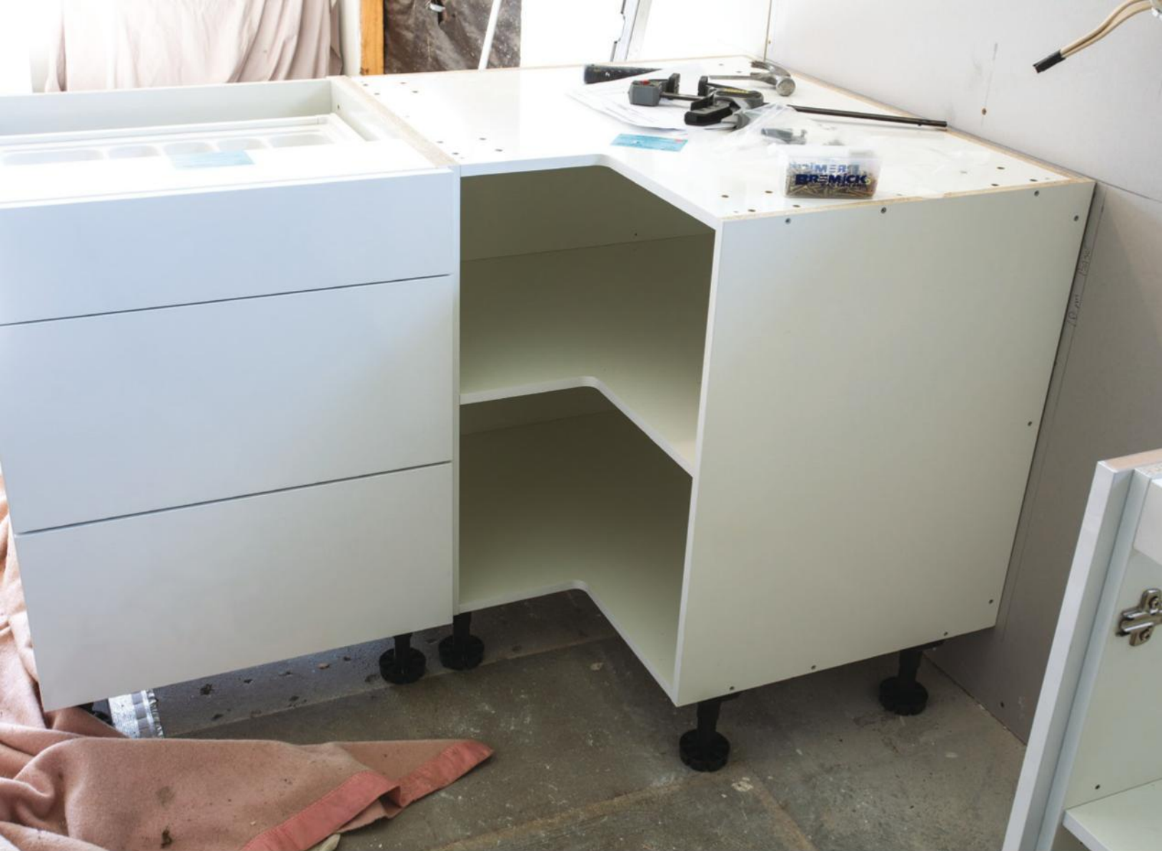
Above and below: The cabinetry for this install was assembled on-site, but sometimes off-site is a good option
