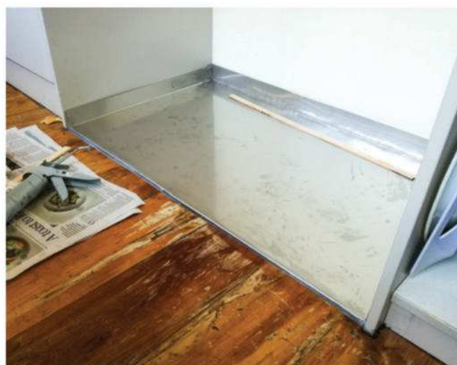
Finished base in place — I sealed the back corners and the slot along the front with Sikaflex 291
