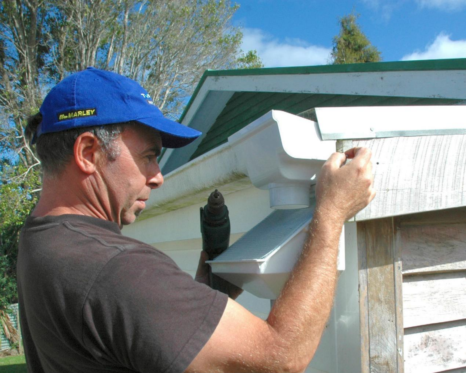
Above: Attaching a rainhead
