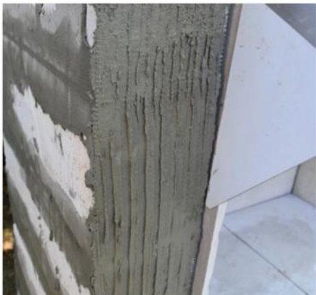
The scratch coat on perimeter around stainless and refractory components
