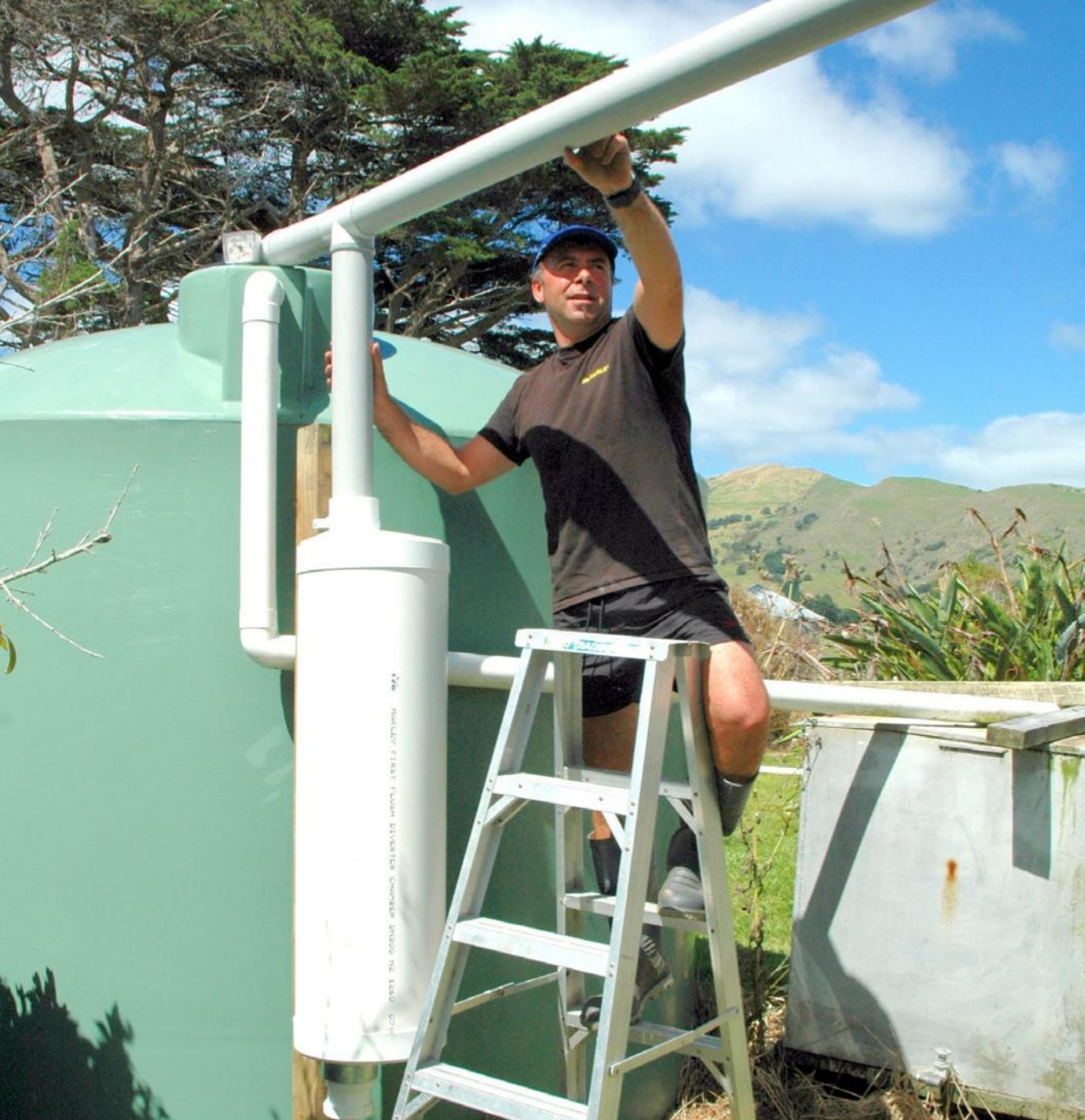
Attaching the first-flush diverter
