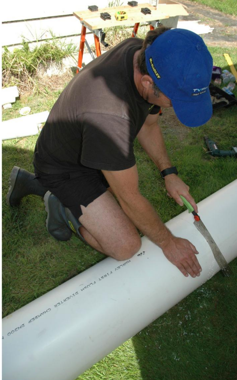
Above: Cutting 300mm pipe for the standalone diverter
