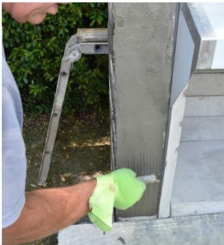
The scratch coat on perimeter around stainless and refractory components
