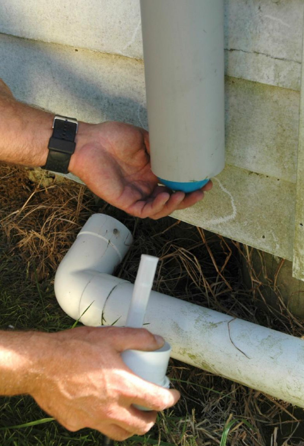
Above: Showing how the ball valve works blocking the diverter
