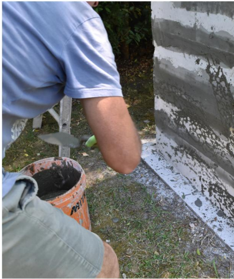
Above and below: The flick coat can be applied with a cut down block layer's trowel
