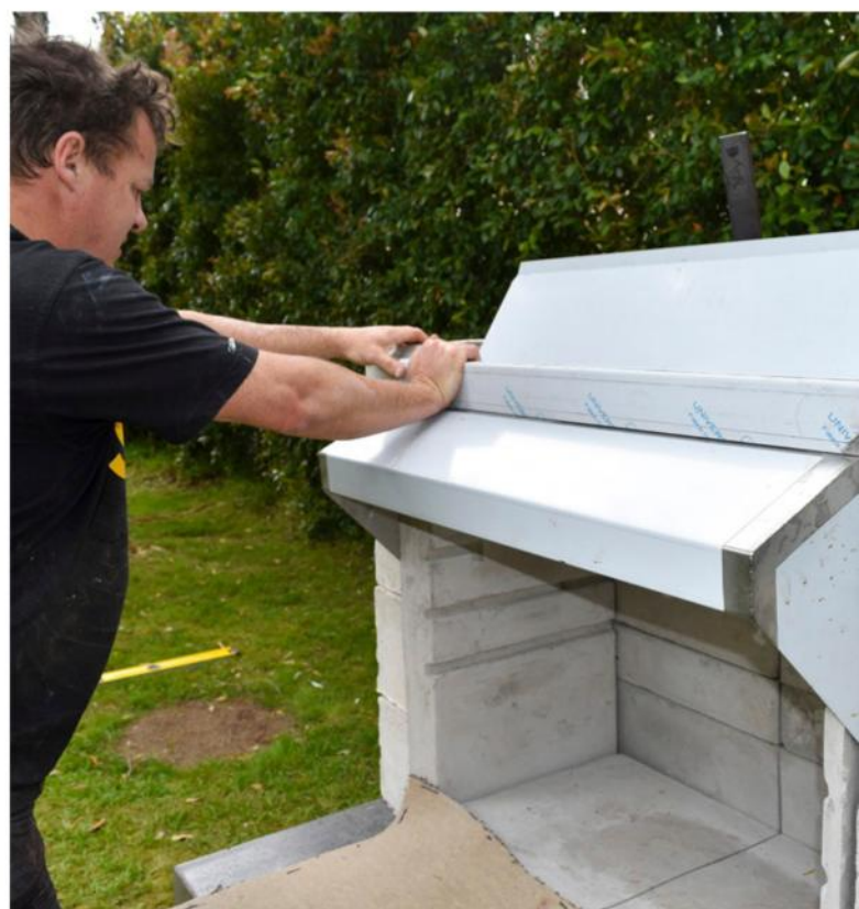
Below: The gap between the firebox and the outer bricks is filled with scoria to act as insulation
