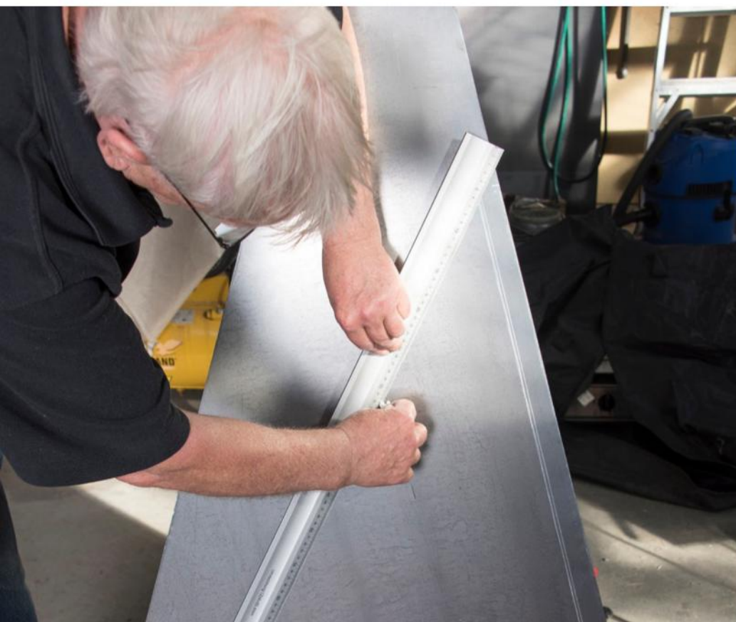
Marking the cut-out for the front
