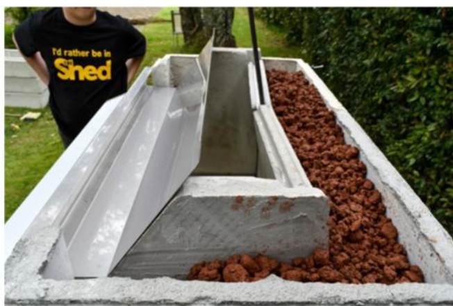
Below: The gap between the firebox and the outer bricks is filled with scoria to act as insulation
