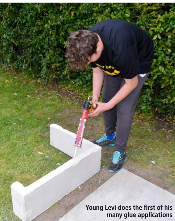
Bottom layer getting positioned on the pad
