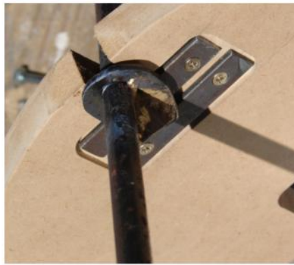
... so the turned up end fits neatly between two steel strips screwed to the underside of the step
