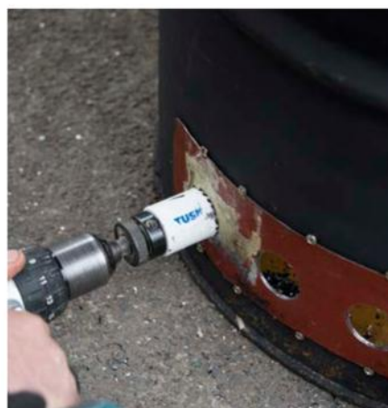
Cutting the holes in the damper
