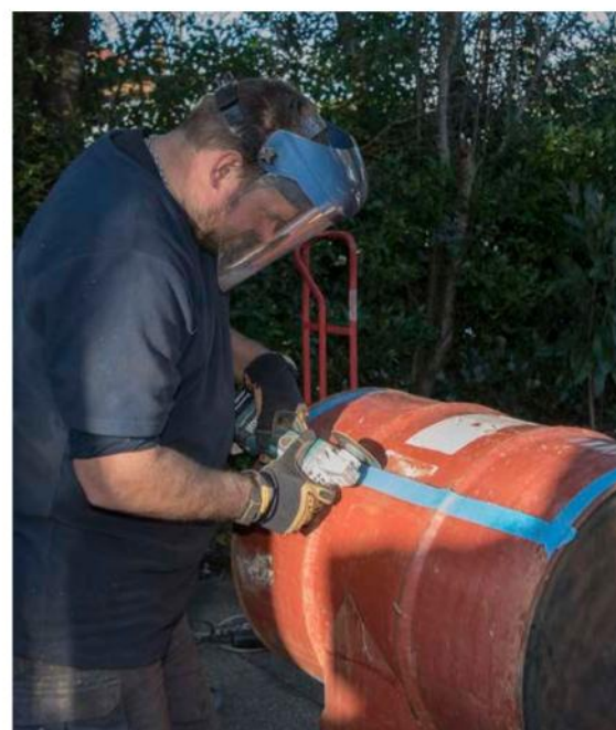
Cutting the back of the door
