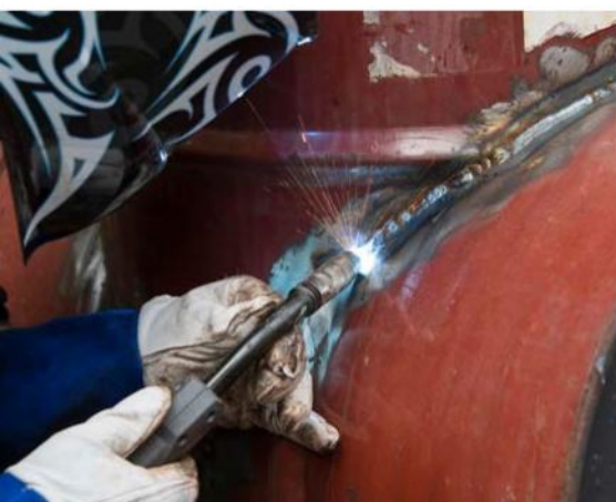
Weld in short runs
