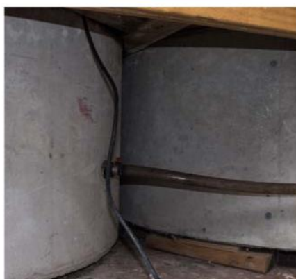
Behind the façade – the tanks, return hose and step-down transformer
