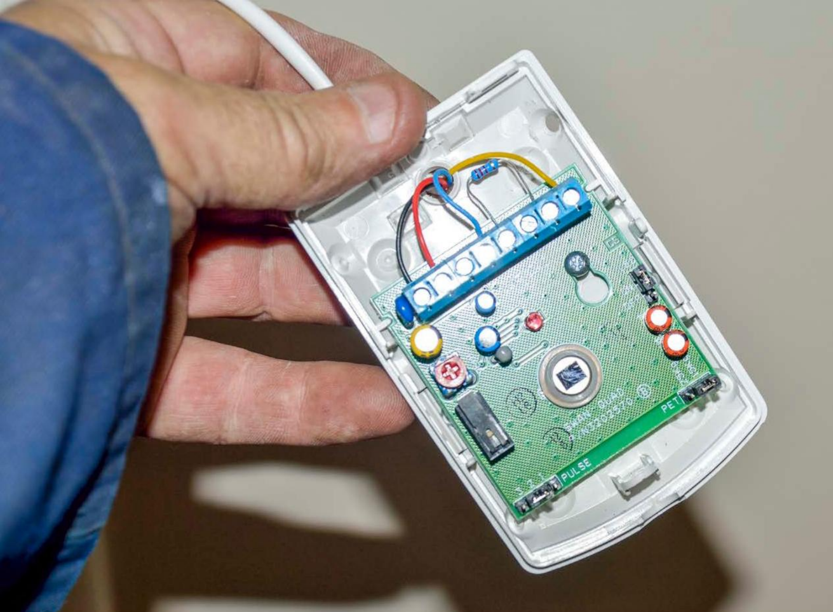
Wiring the PIR at ground level then fitted in the corner leaving clearance at the top
