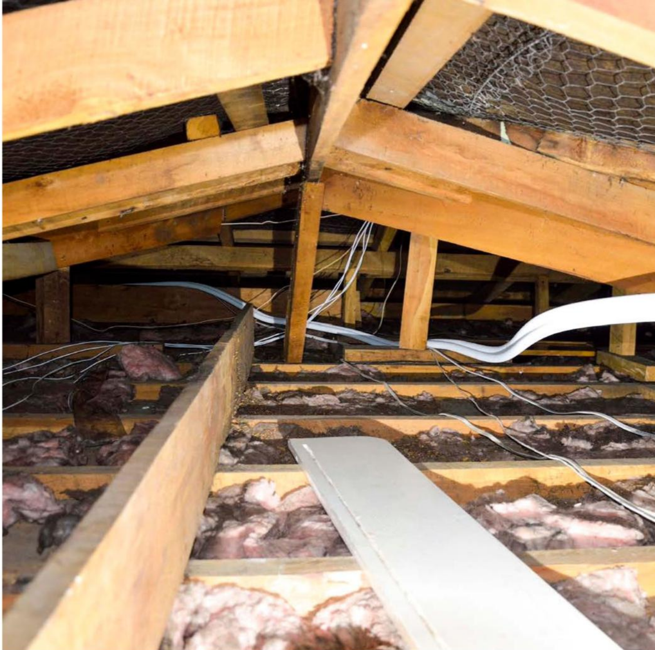
Above: Showing low roof pitch and unsupported air conditioning pipes by 'professional installers'
