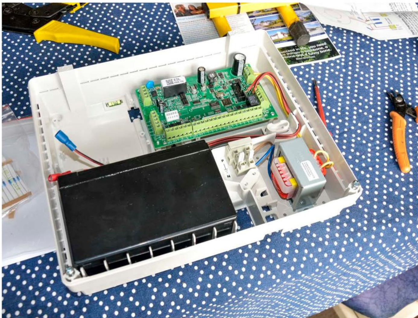
Wiring battery lead before fitting and terminating cables
