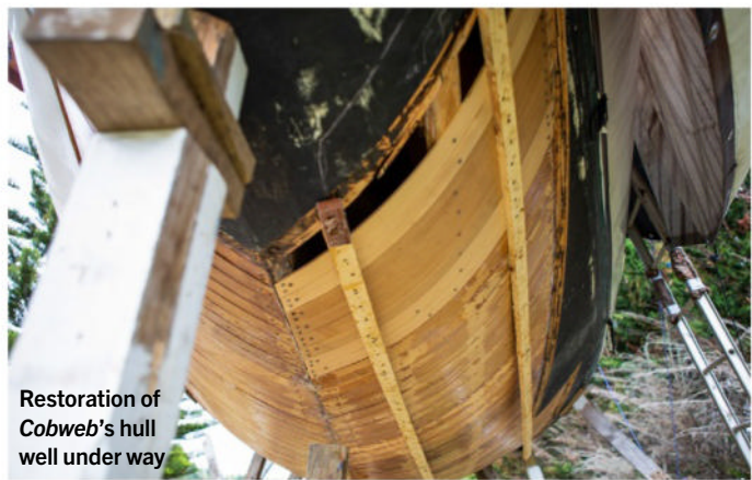
Matt stripping out Cobweb's hull
