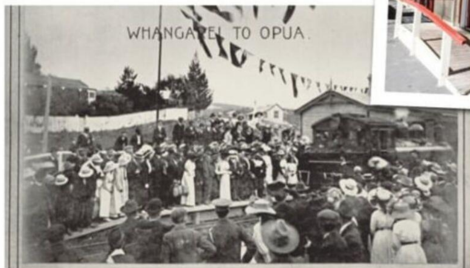
THE COMPLETION OF ANOTHER LINK IN THE NORTH AUCKLAND RAILWAY SYSTEM.
