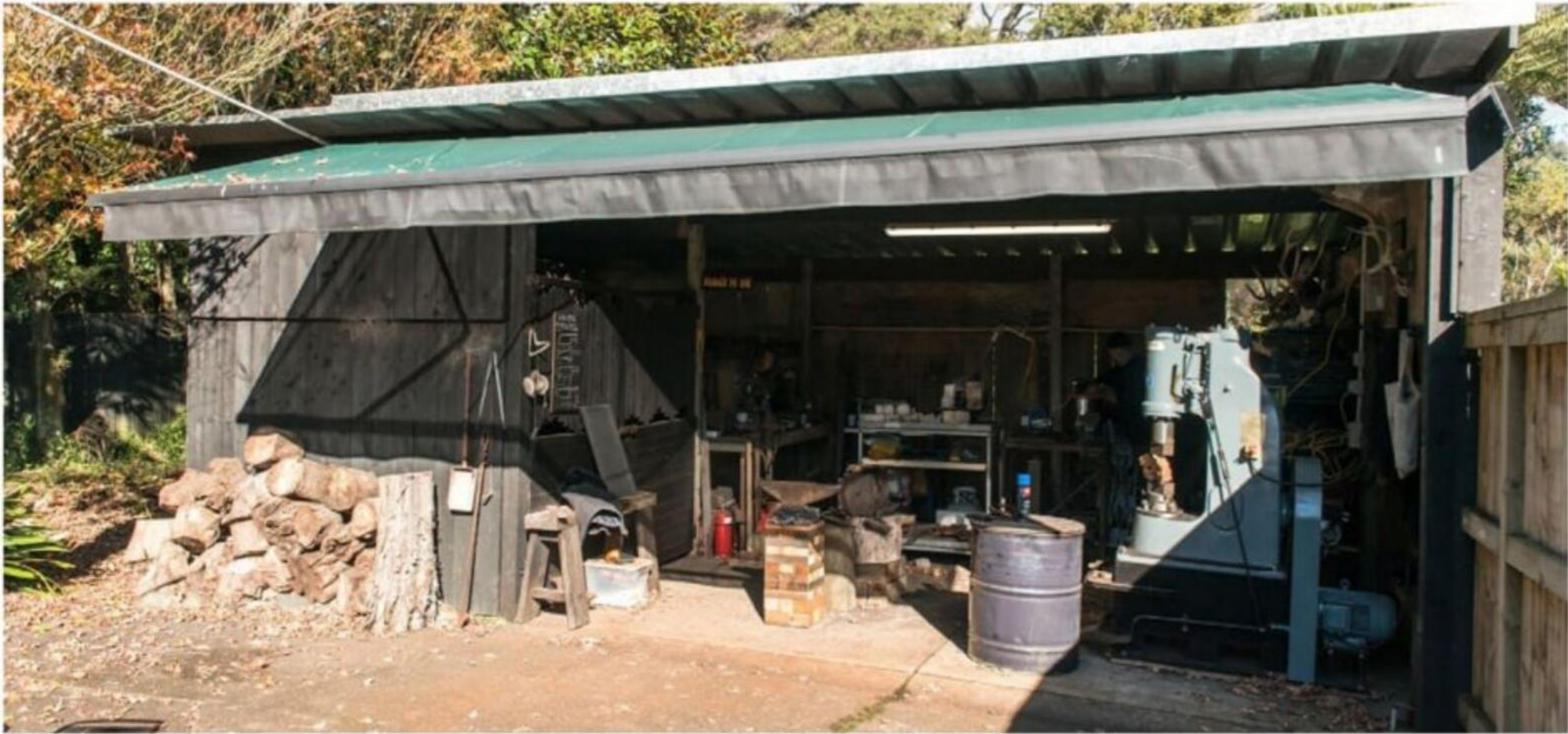
The forge shed
