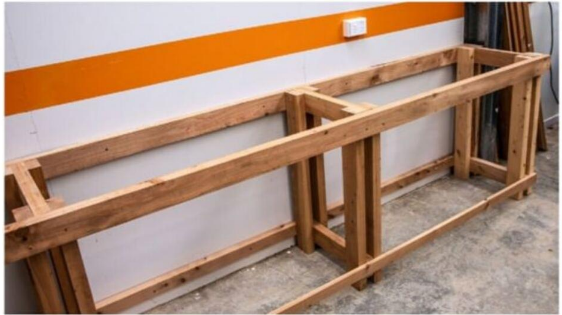
The frame in place
