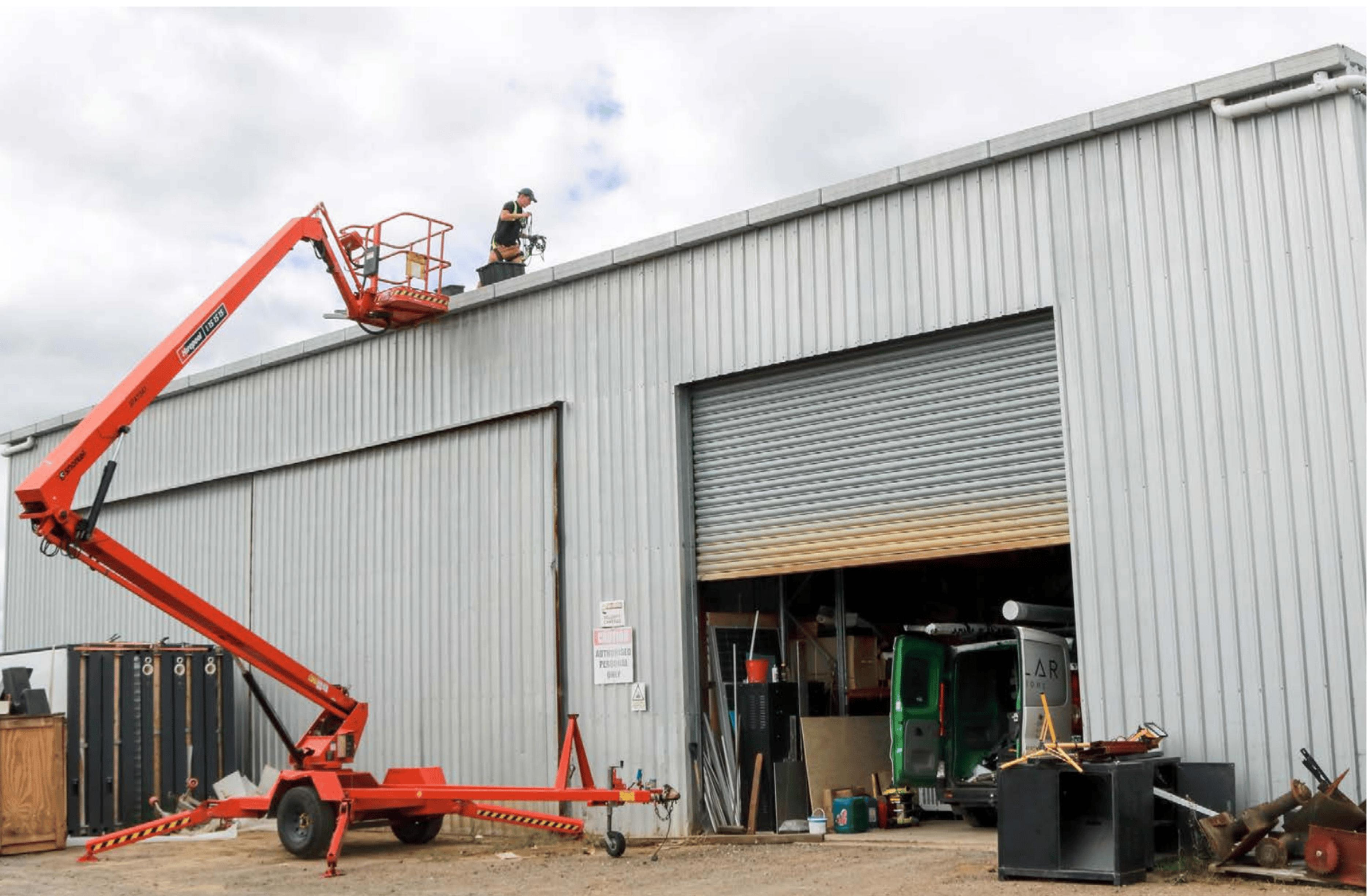
An added cost was a scissor lift to get the 32 panels and all the railing up to the top of a 6m stud shed. Weather is a factor here; you don't want to be installing 2x1m solar panels if it's windy
