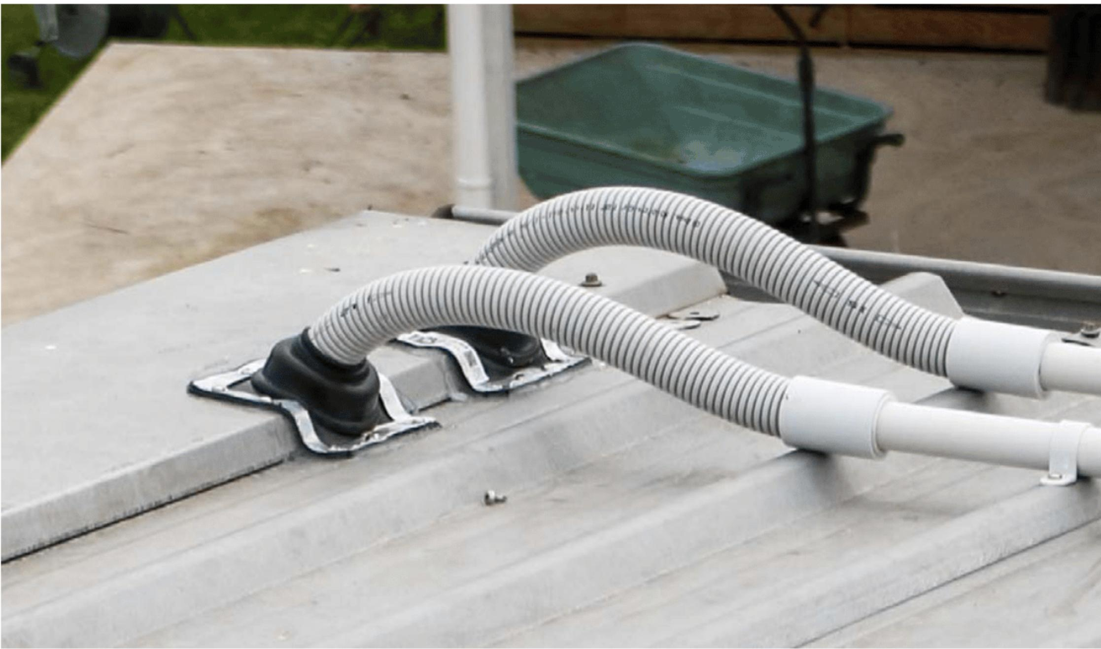
The roof penetration fittings for the electrical feed from the panels into the shed. High voltage and lots of electrical current should not be mixed (it's also a metal shed)
