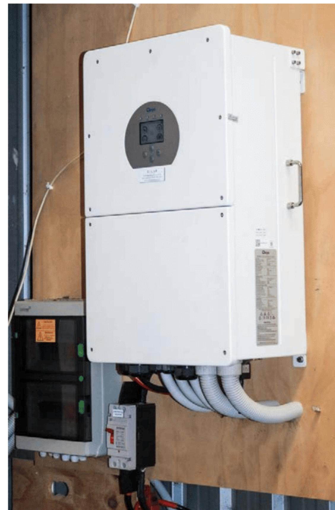
**The heart of the system – a 12kW Deye hybrid inverter**
