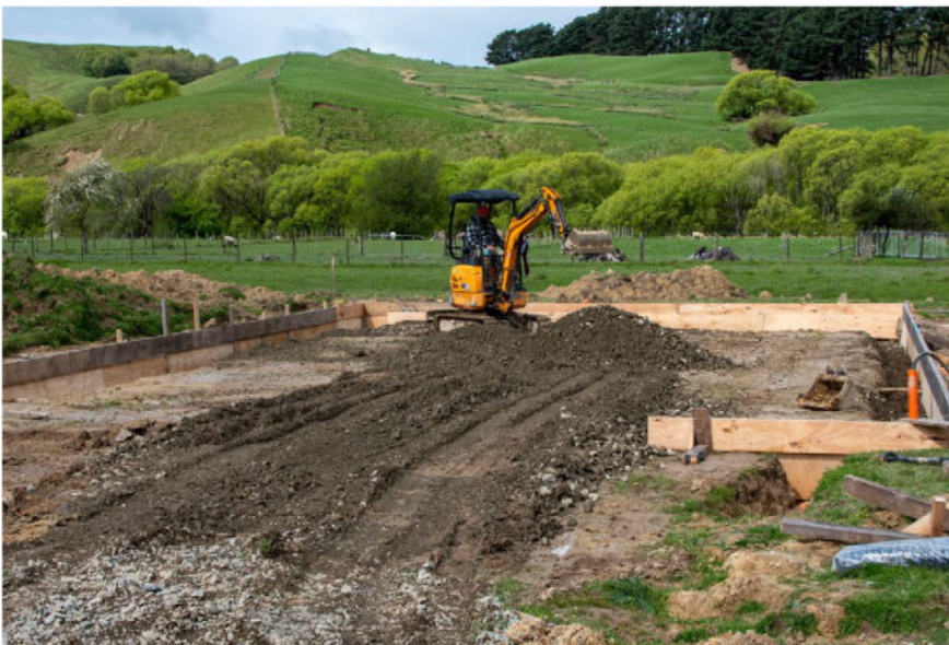
Spreading the base rock. The day after this photo was taken, in early October, it snowed
