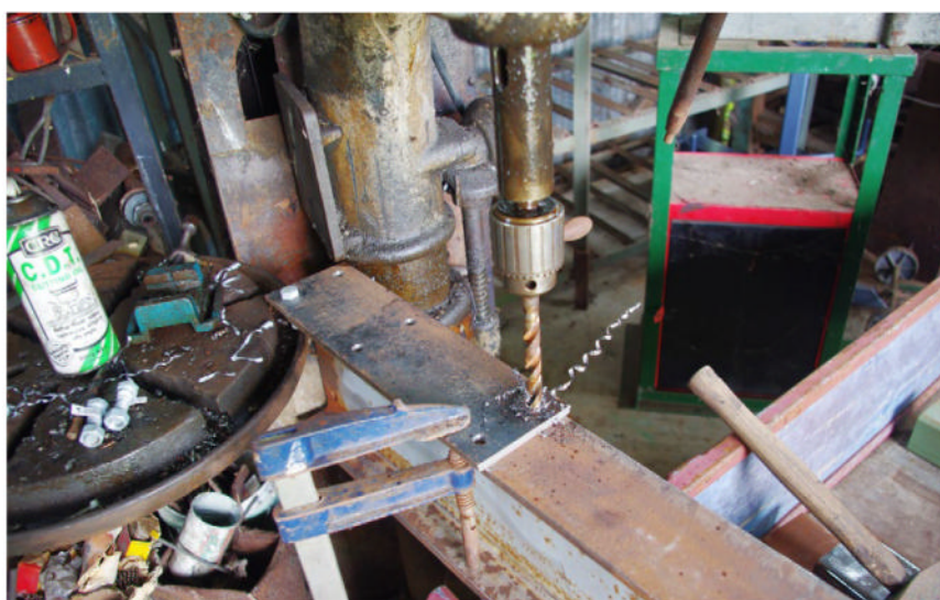
Stanchion plate drilled on I-beam to match
