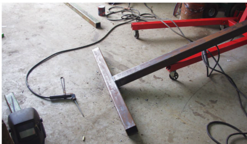
T-bar welded on square
