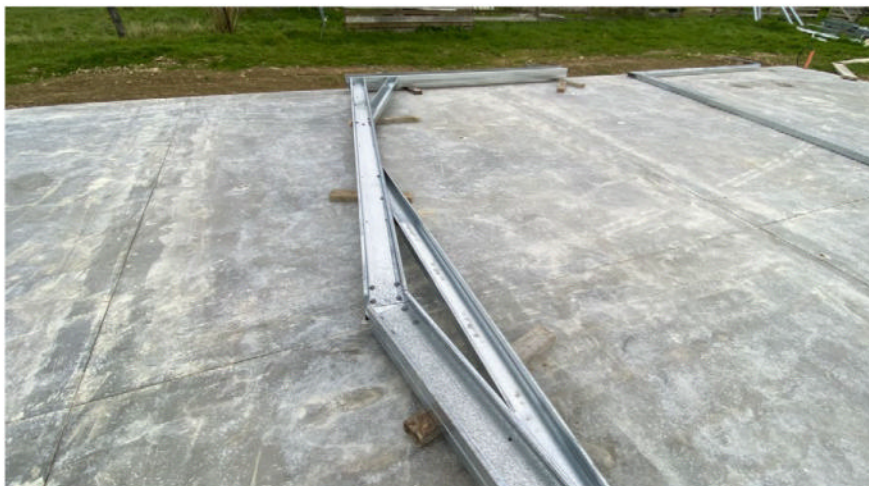
The portals being assembled on the pad
