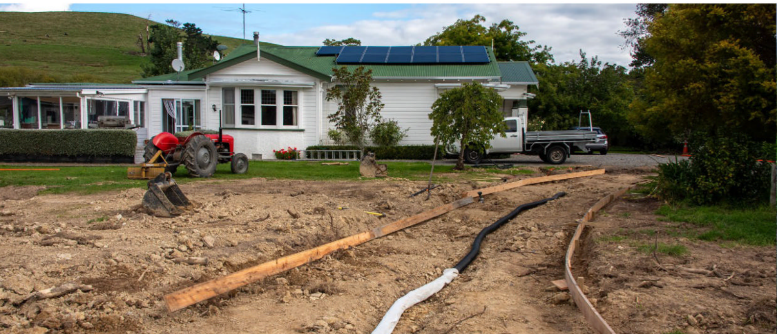
Boxing the road and adding a drain
