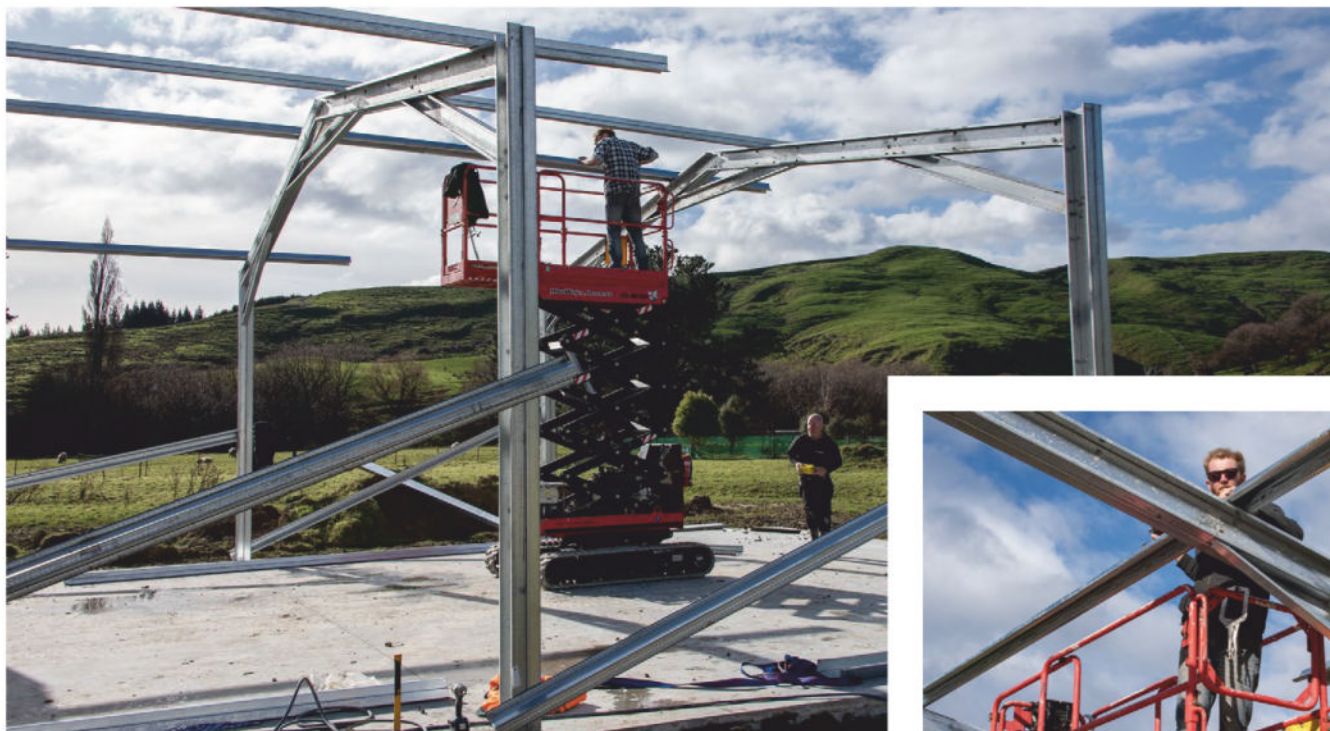
With the help of Andrew and my friend Brian Hill, we made serious progress and had the portals up in two days, along with the purlins installed
