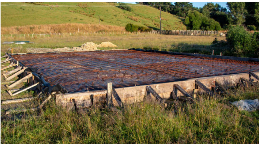
By January 2024, the foundations were finished, the damp course and steel tied and in place
