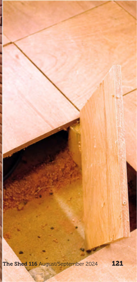
Specially designed concrete-filled pillars to support heavy machinery in the workshop. The floor can be lifted to look after the ducting
