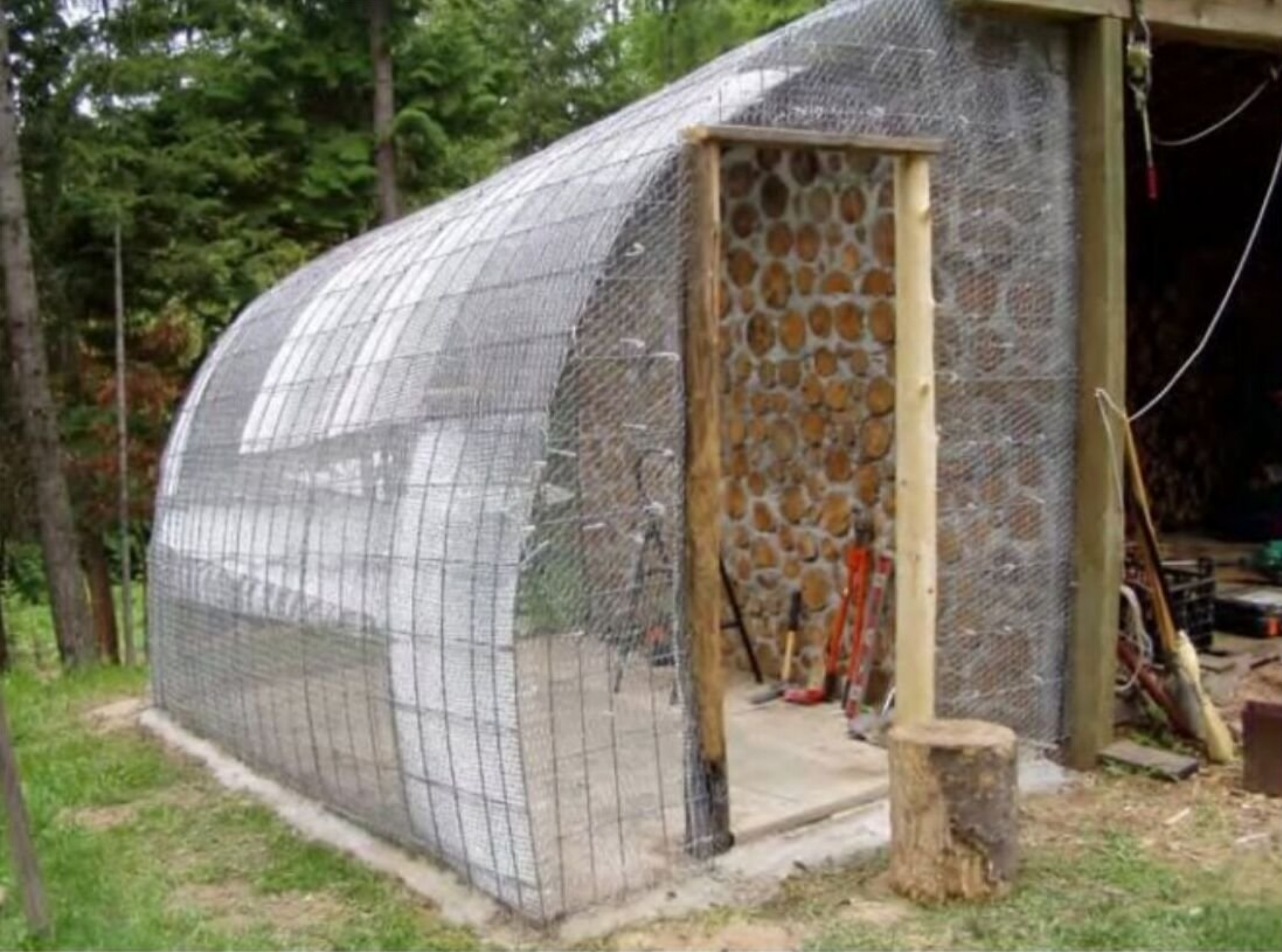
Ties everywhere! Of course, the long tails were cut off before plastering
