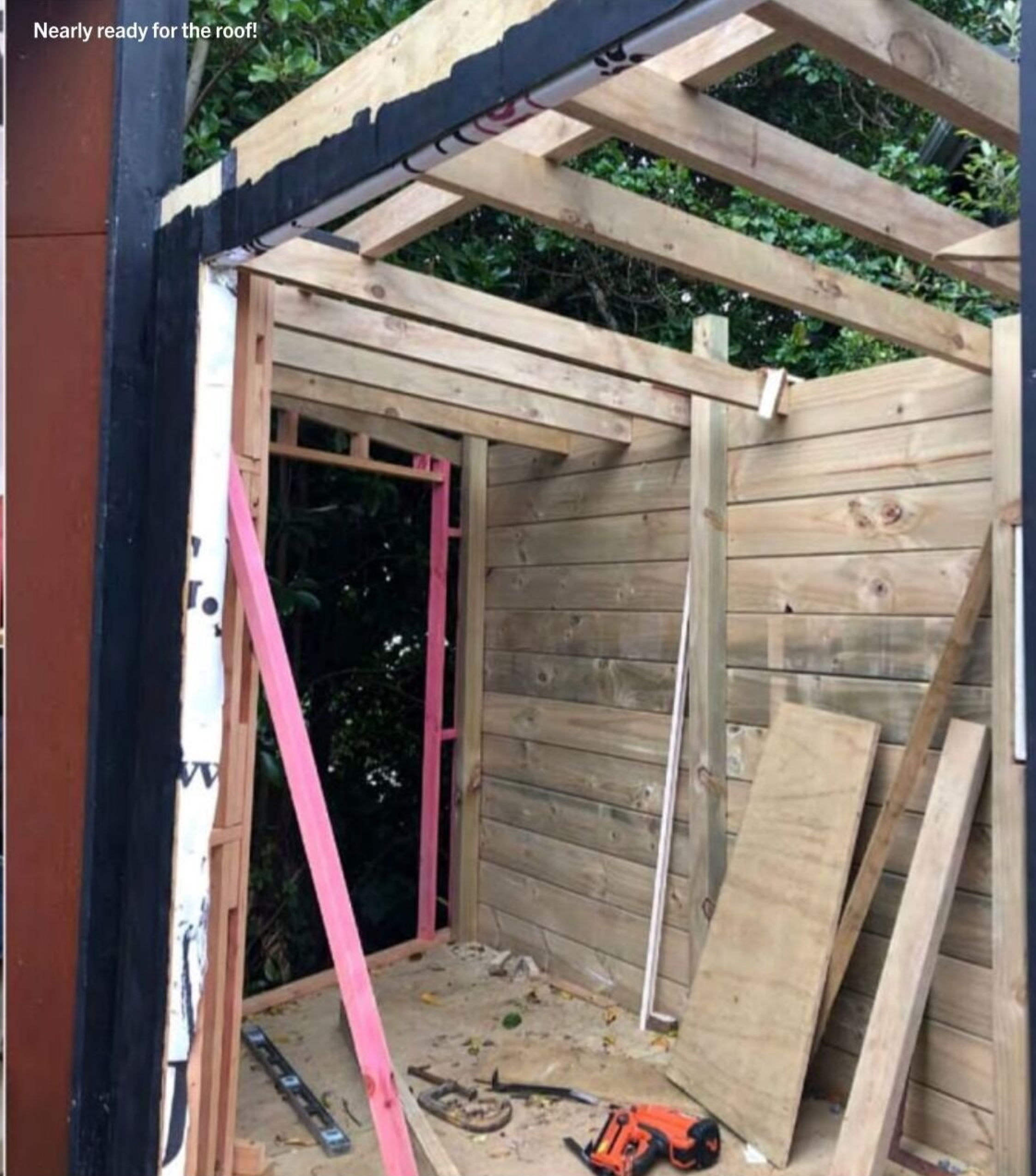
Cousins helping to screw down the roof
