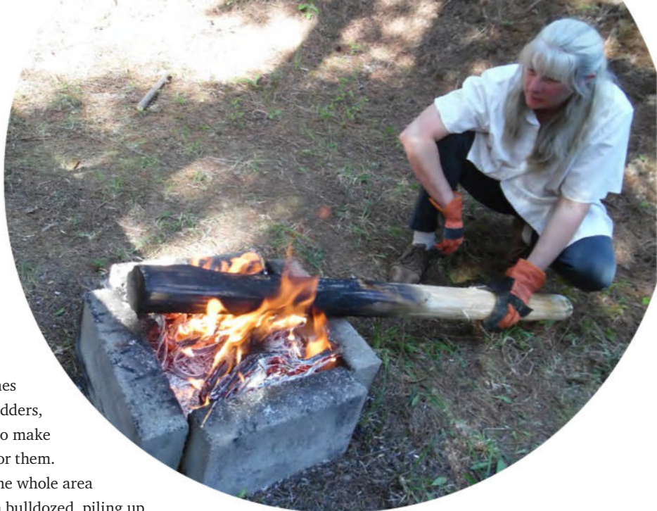
We preserved the ends of the uprights by charring them well in a fire
