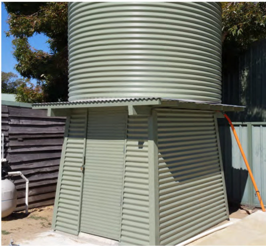
The tank stand is closed in as a small, detached shed for storing dangerous materials
