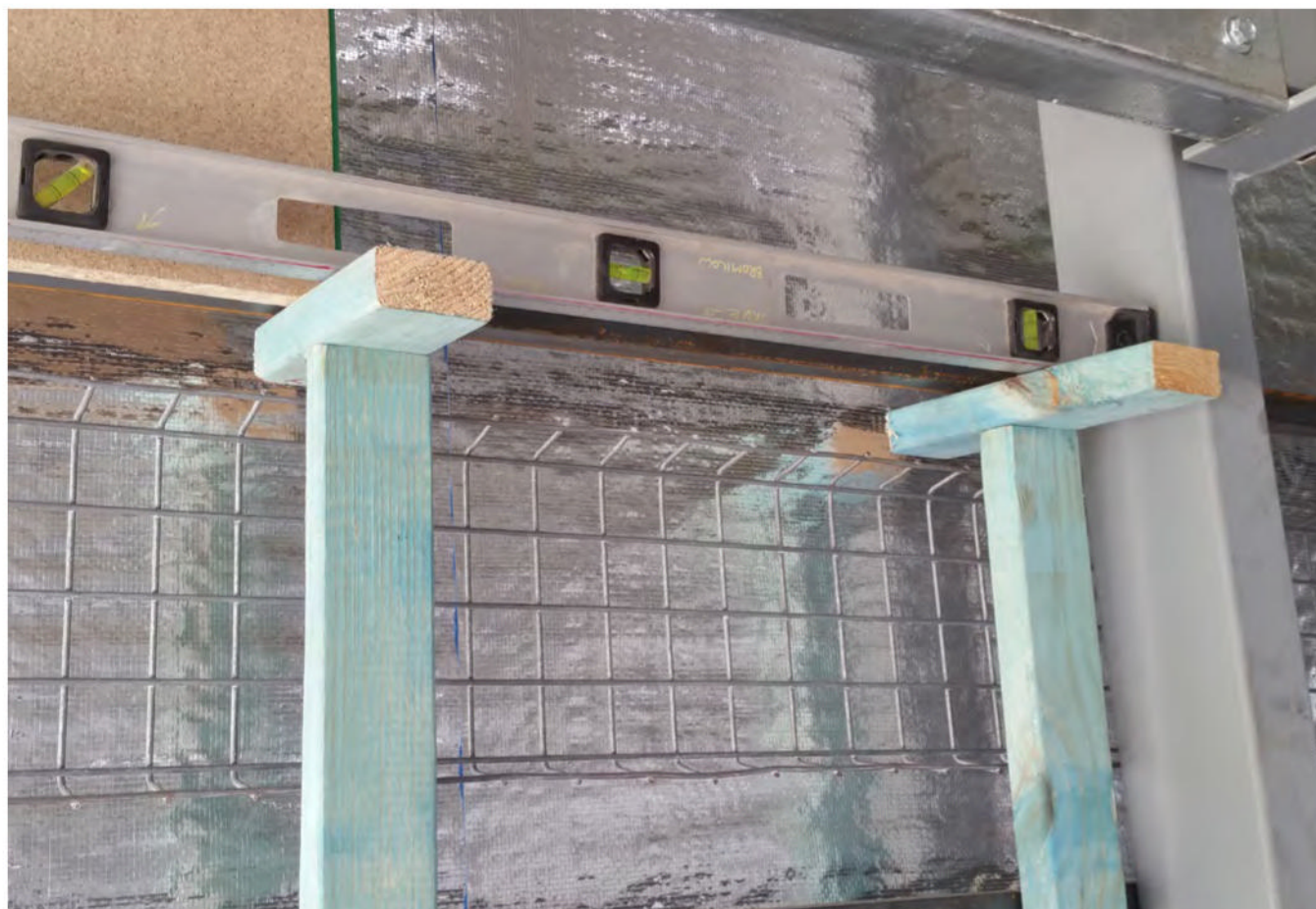
Below: Photo 15 – The sheets were supported from the bottom on a pair of temporary stands
