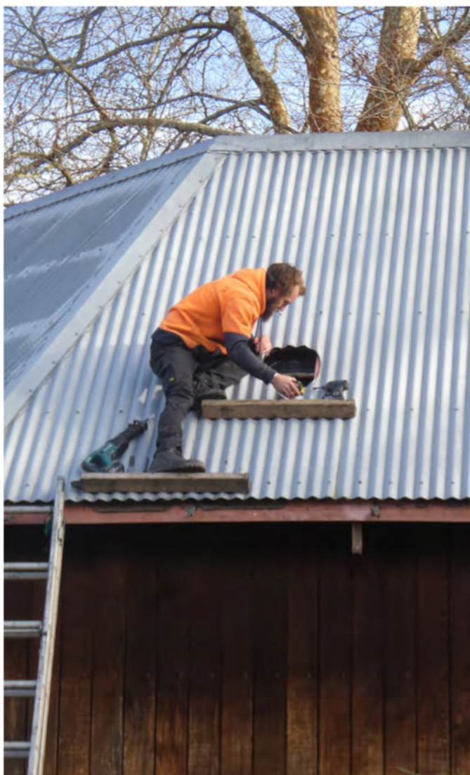
Completed roof opening — the wooden framing assembled inside the roof is just visible
