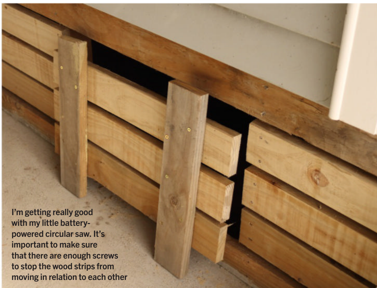
The finished door — it won't be used often, so it isn't hinged. The piece of wood sticking out the bottom sits on a strip behind the lower board to line up the door when fitted. A strip of wood on the inside framing on each side stops the door from falling inwards
