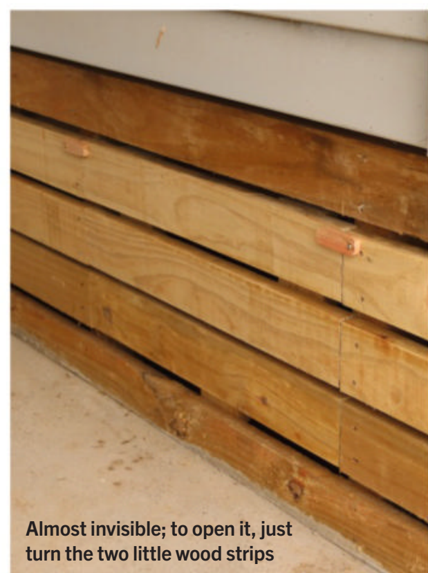
The finished door — it won't be used often, so it isn't hinged. The piece of wood sticking out the bottom sits on a strip behind the lower board to line up the door when fitted. A strip of wood on the inside framing on each side stops the door from falling inwards
