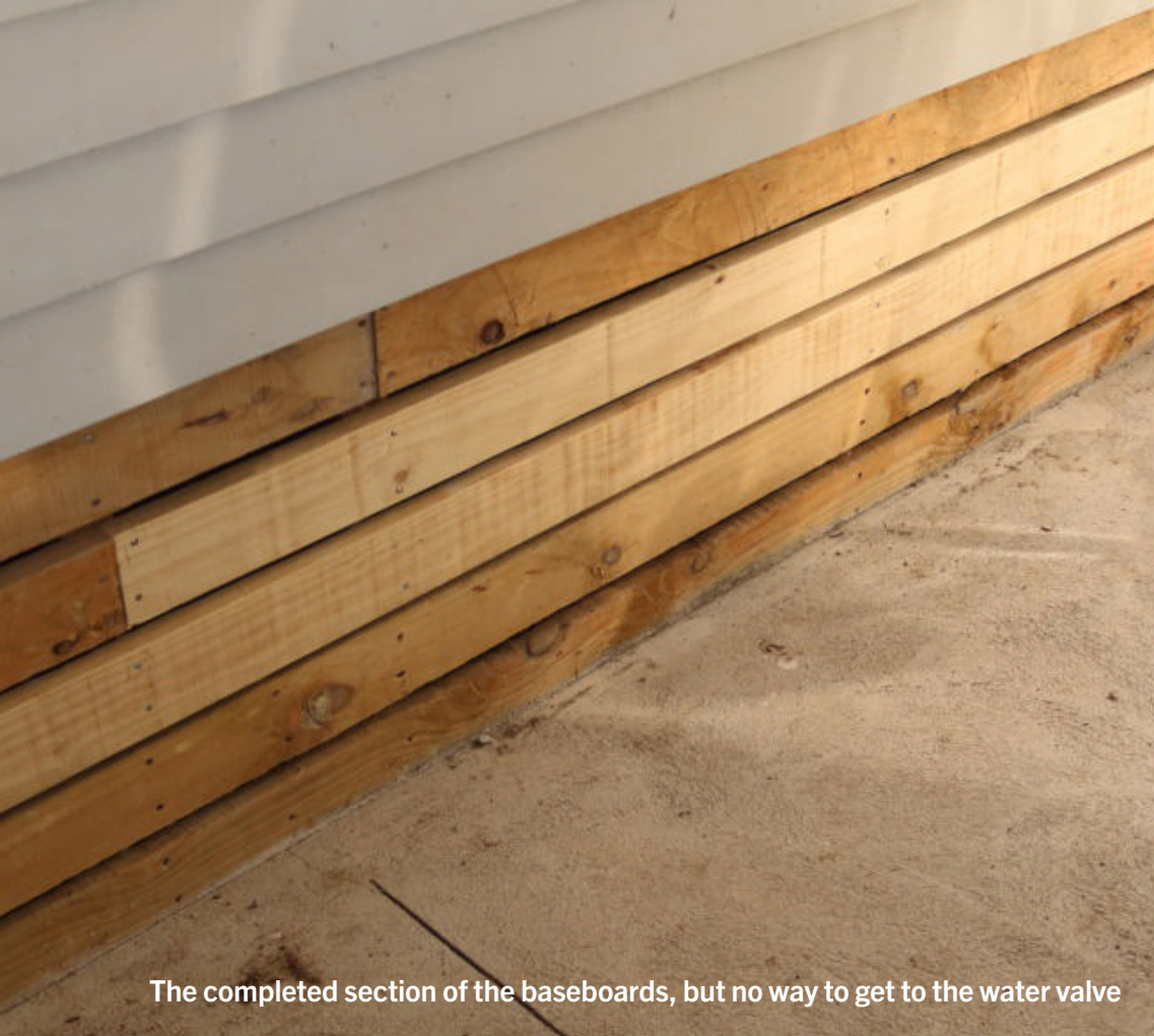
First, I marked where the door was going to be on the already-fitted baseboards. The lines run down the inside of the two internal bits of framing. It's a good idea to screw on some temporary boards to hold the boards that you are going to cut through in place once you have cut them free
