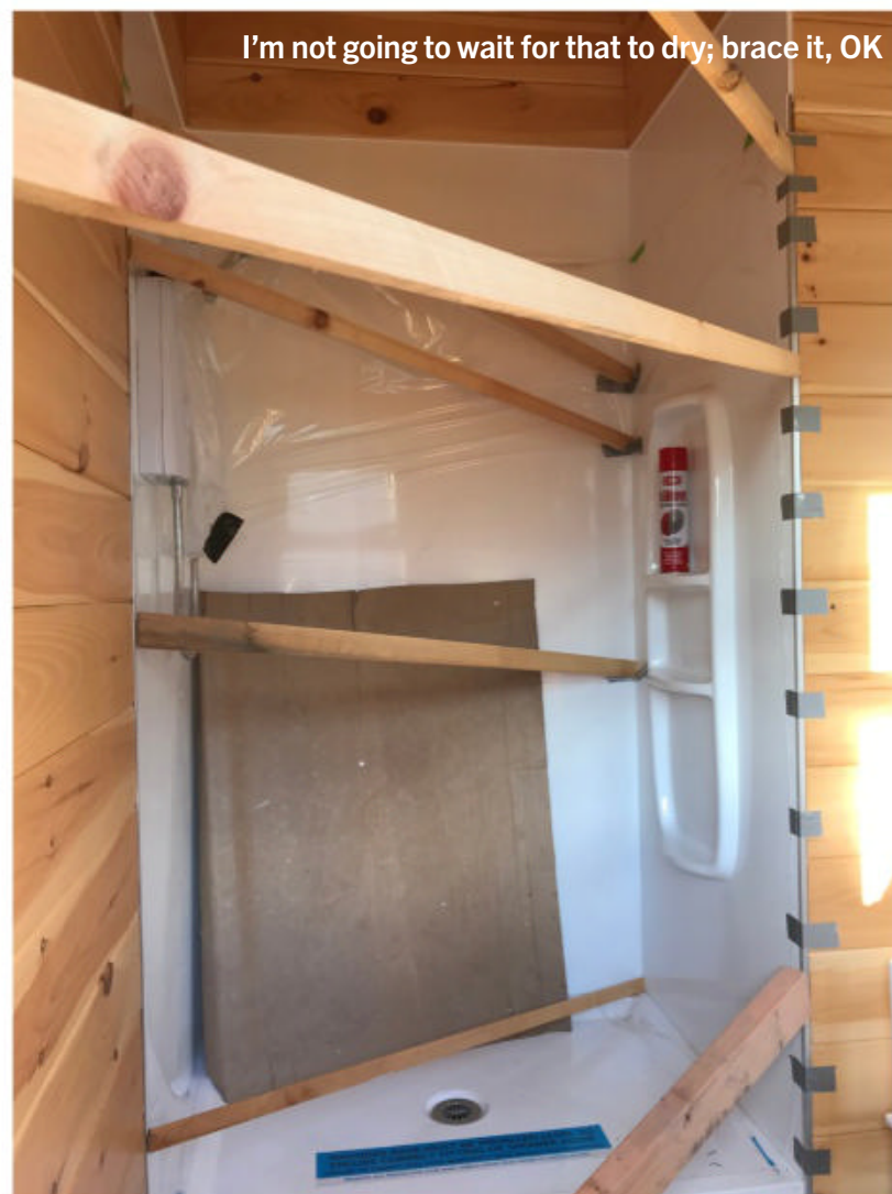
Master bedroom and en suite in progress
