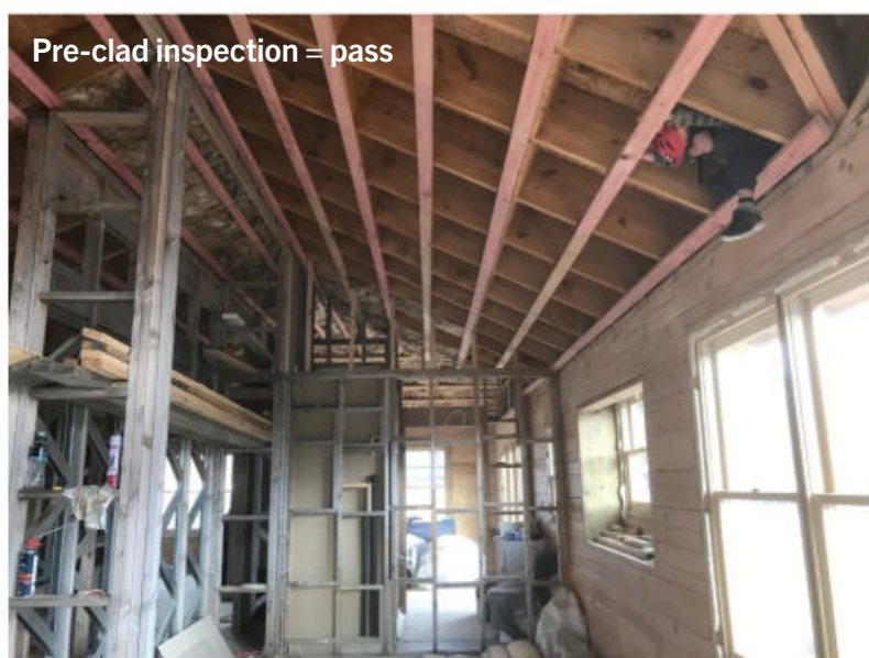
Master bedroom — knee-wall plus bracing
