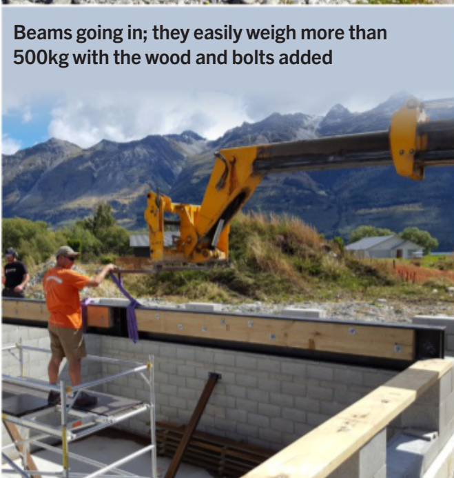
More beams — note the 45-degree braces I welded and bolted to the walls to enable 100 per cent of the backfilling to be done
