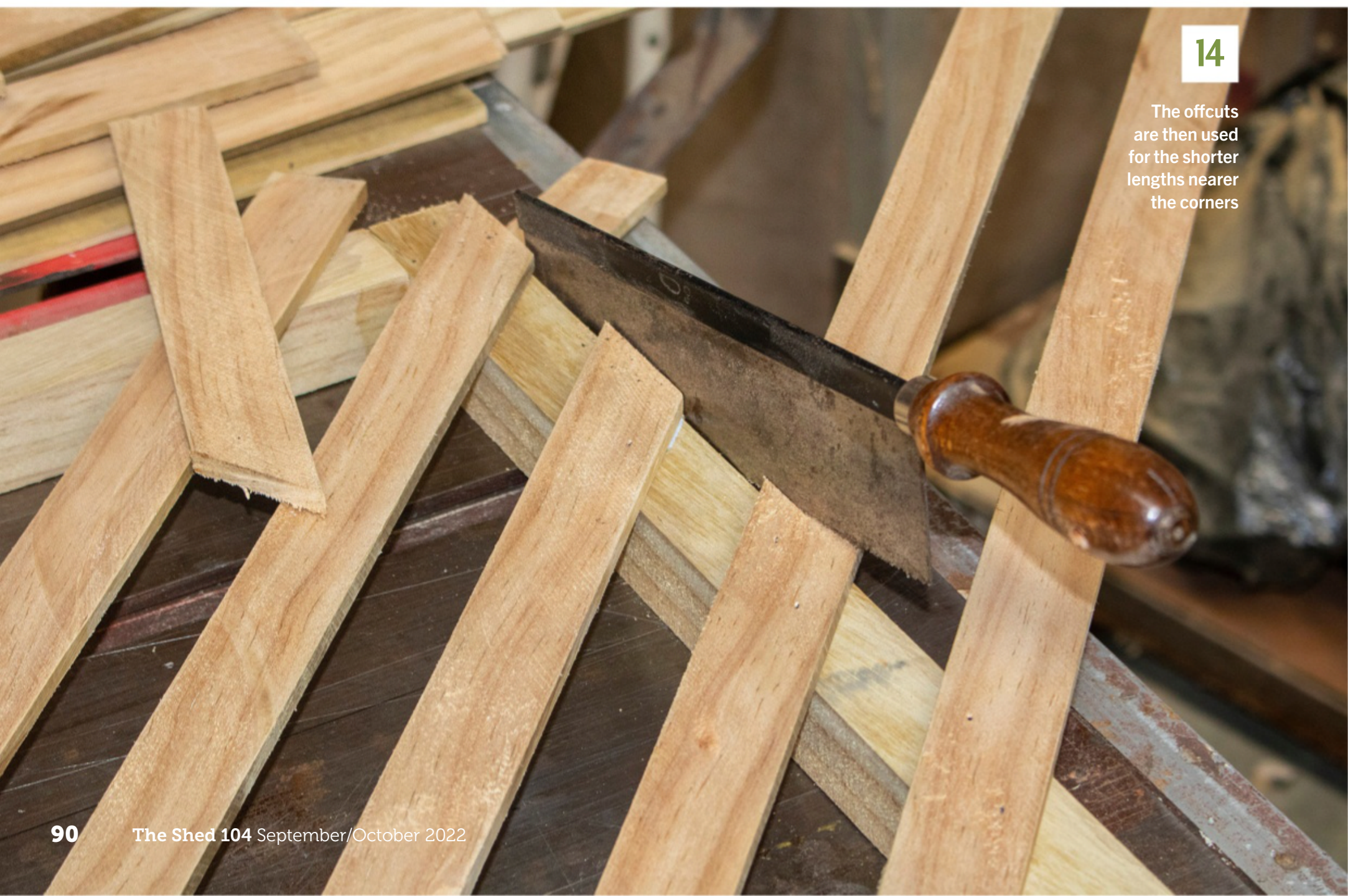
Note the overhanging strips. These are cut off using the edge of the frame as a guide
