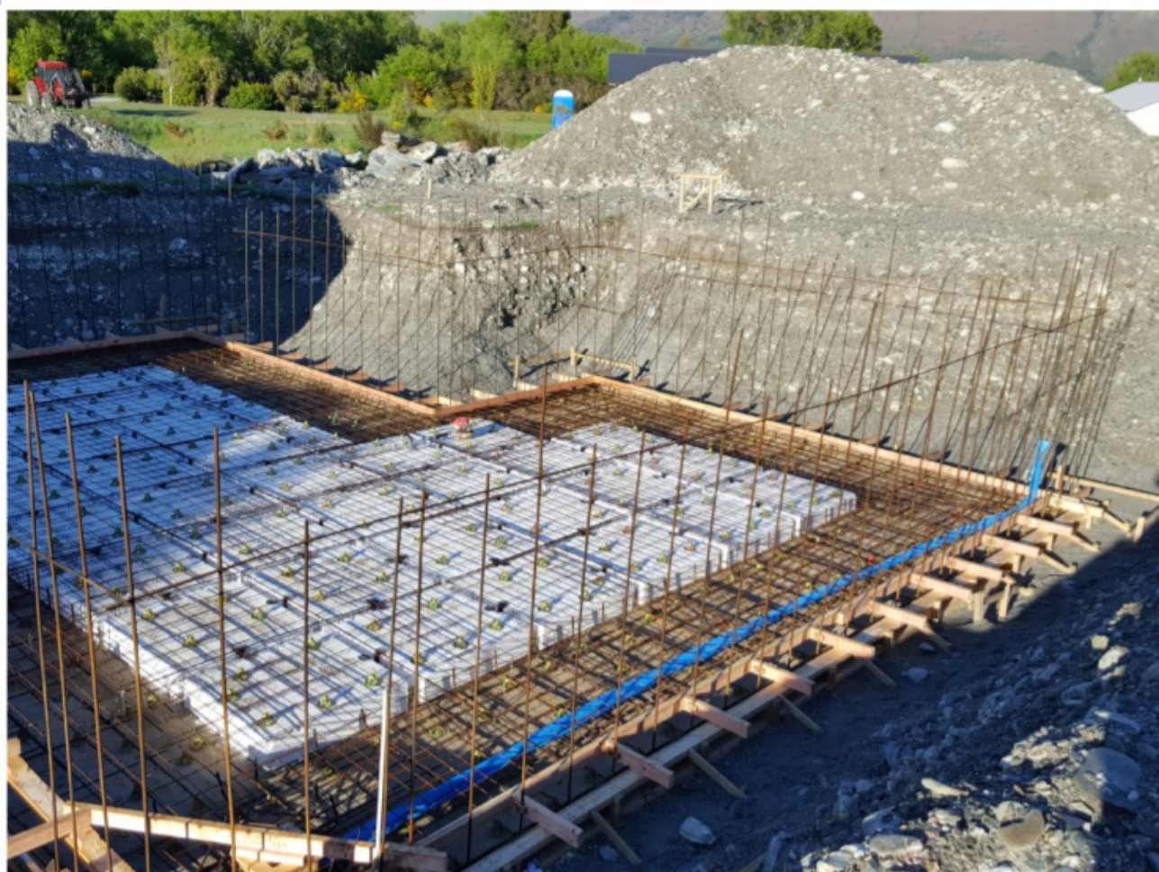
Left: The finished foundation after busting my ass for 36 hours straight — awaiting concrete
