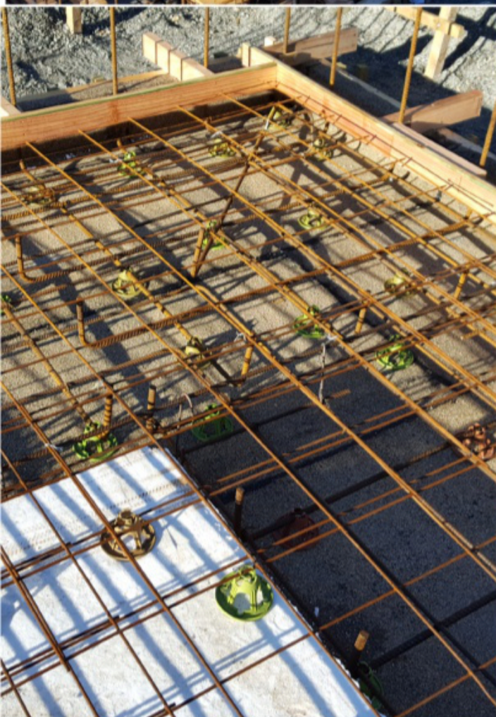
Corner detail; neat as you like as far as laying rebar goes
