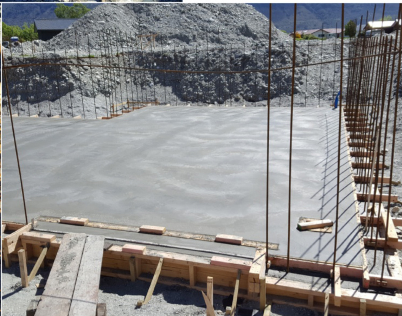
The finished pour; wood covers the drain inside the door which will eventually have a float-activated sump pump
