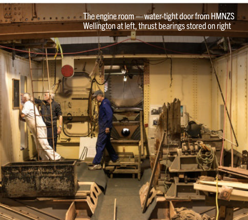
Grinding underway to prepare rib V-butt joints for welding
