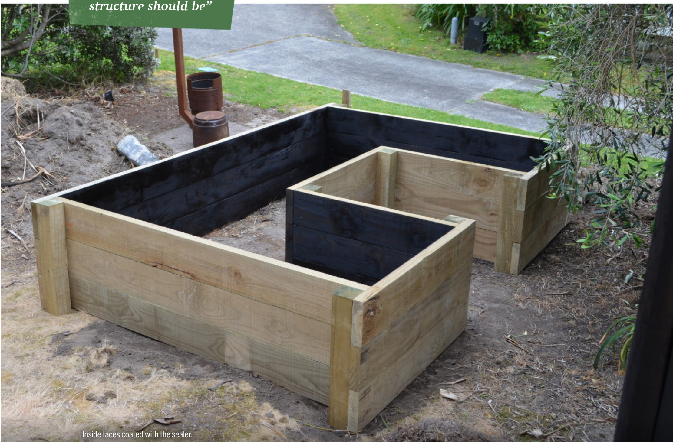
Side boards all on
