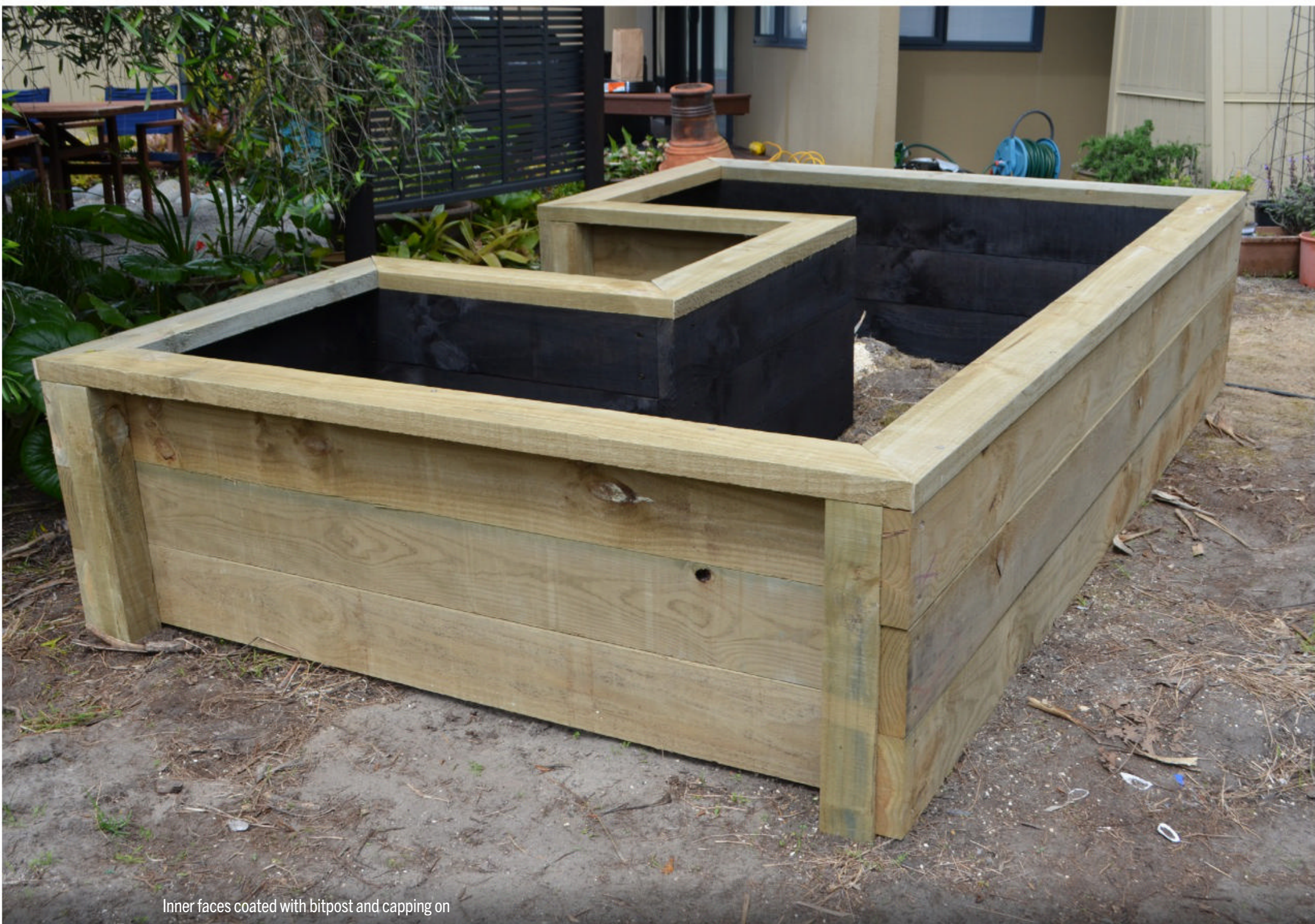
Mitred join at the ends of the capping boards
